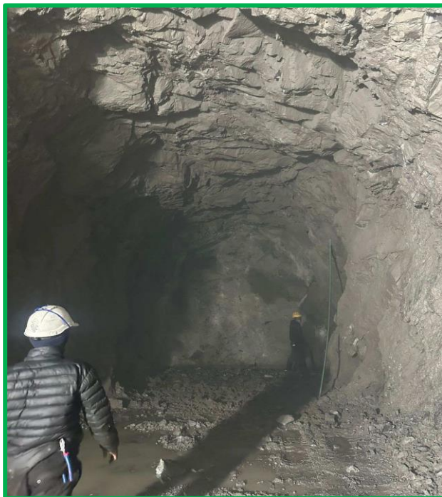
Figure Showing :- Fullface Excavation from Outlet to Slope Breaking Point.
