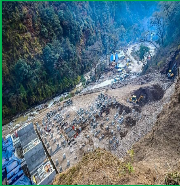
Figure Showing : Completion of Foundation Works at Switchyard.
