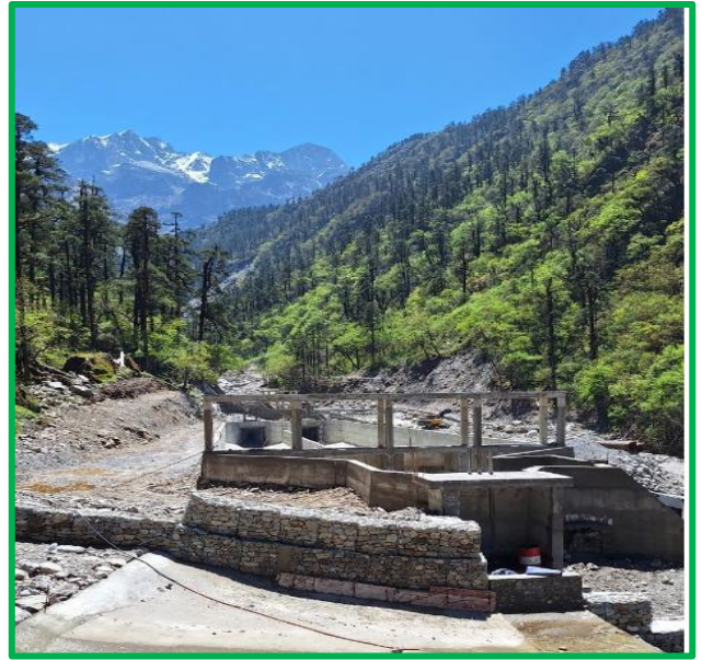
Figure Showing :- Overall View of Likhu Desander at Headworks.
