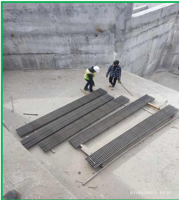
Figure Showing :- Inspection for Fabrication of fine trash rack at Likhu Headworks
