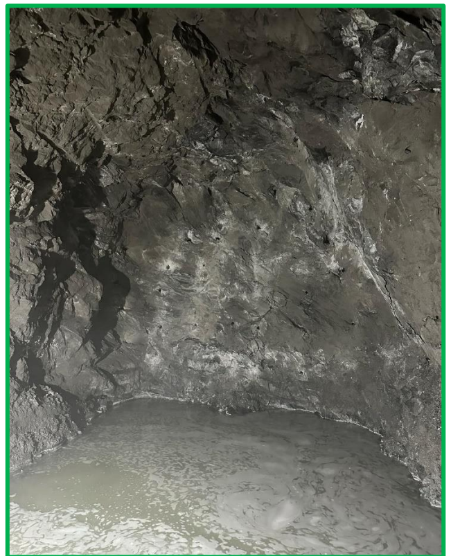
Figure: Tunnel face of NL-junction to Nupche Inlet (F2) at ch: 558.6m.
