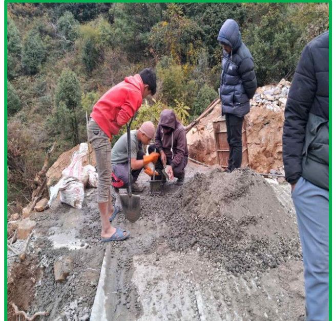
Figure Showing :- Cube casting at site for quality check of manual mixed Concrete.
