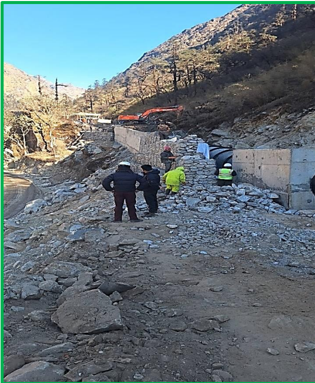
Figure Showing :- Gabion and protection works along Nupche HRP.
