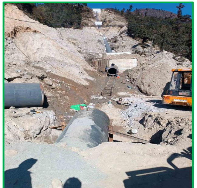
Figure: Concreting of Anchor Block along penstock pipe alignment.
