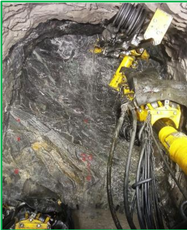
Figure:- Drilling works using Boomer from NL Junction to Nupche Tunnel.
