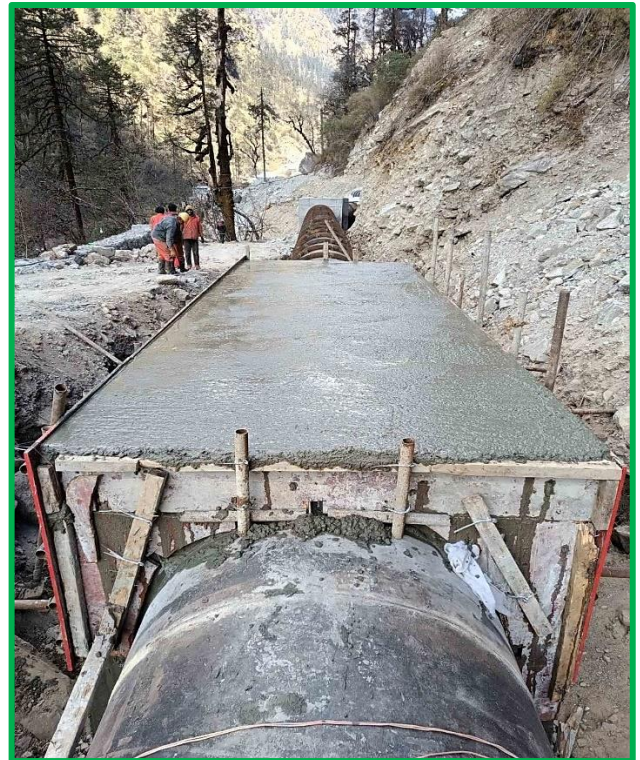
Figure Showing :- Concrete casing works along Nupche HRP
