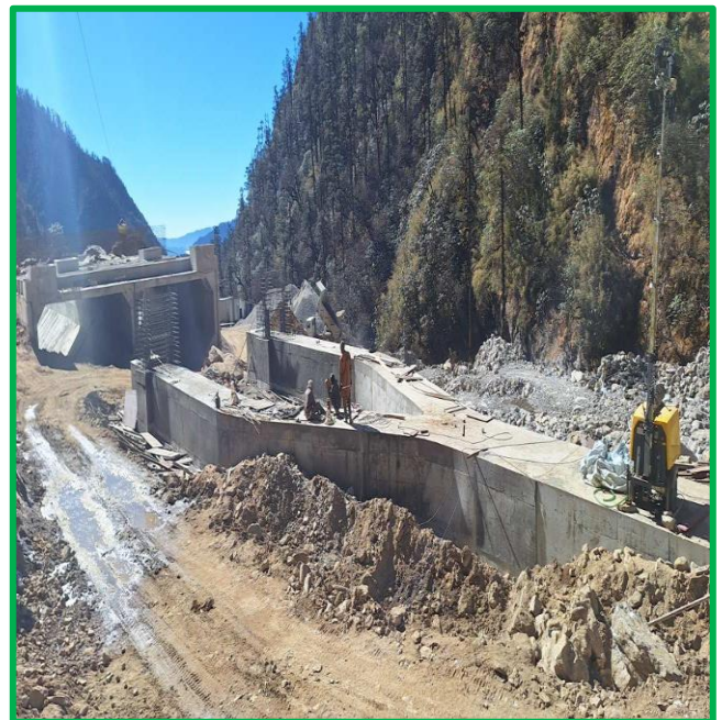
Figure Showing:Completion of Concrete works at Y-section above Gravel Flsuhing at Nupche HWs.
