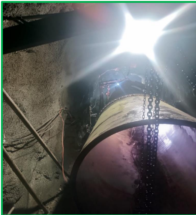
Figure Showing: Erection of pipe at Penstock Tunnel.
