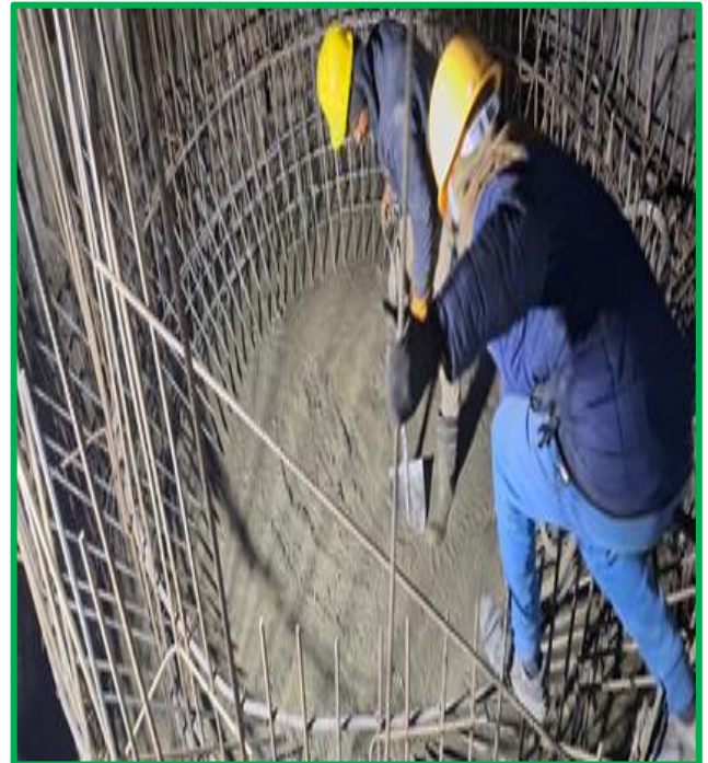
Figure: Concreting Works started at Surge Shaft.
