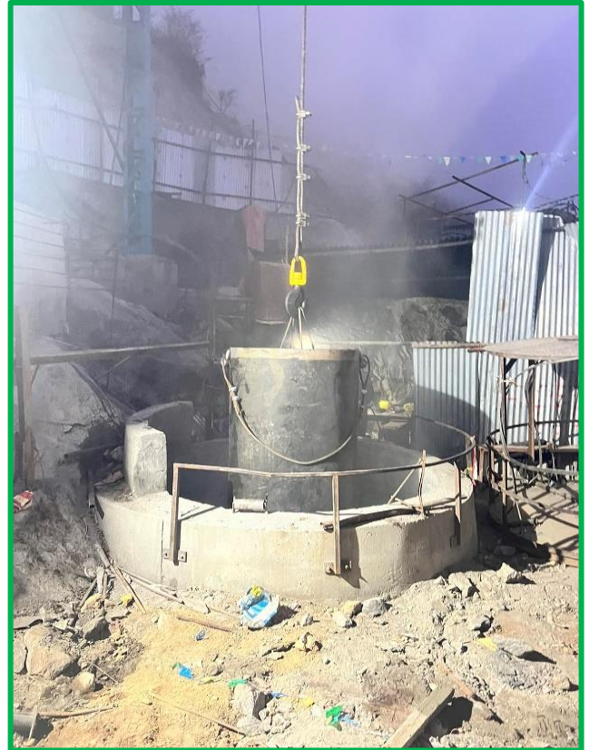
Figure Showing :- Lowering of Pipe at VT.
