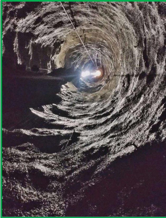
Figure Showing :- Vertical Shaft (Full Face).
