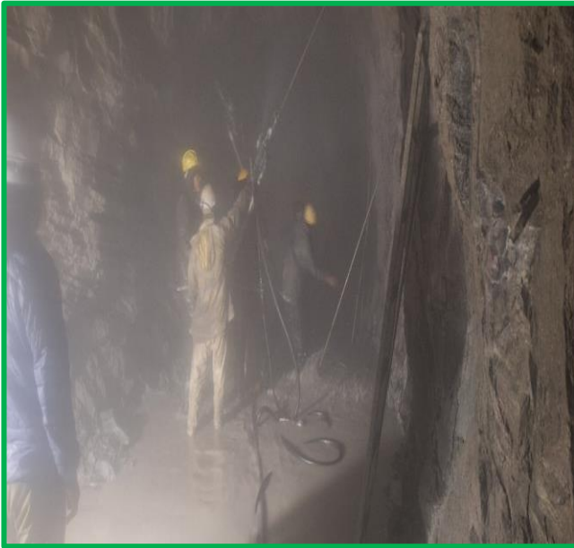
Figure Showing :- Installation of Rock Bolt at Face-2 as tunnel support works
