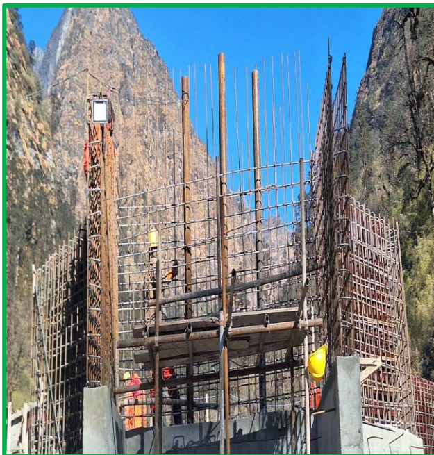
Figure Showing : Rebar works & Installation of Air Vent Pipe Installtion at Headpond Area.
