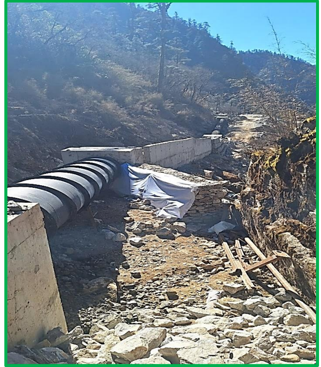
Figure Showing :- Concrete casing works along Nupche HRP
