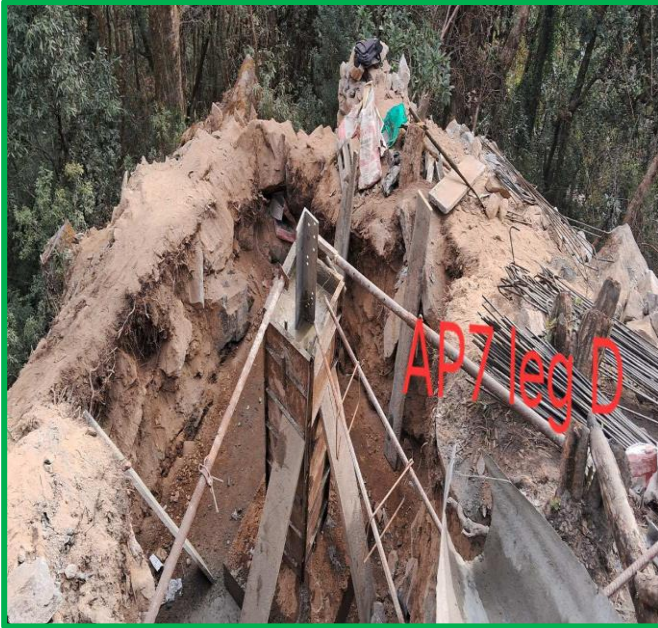
Figure Showing :- Stub Setting and Chimney concreting of AP-7.
