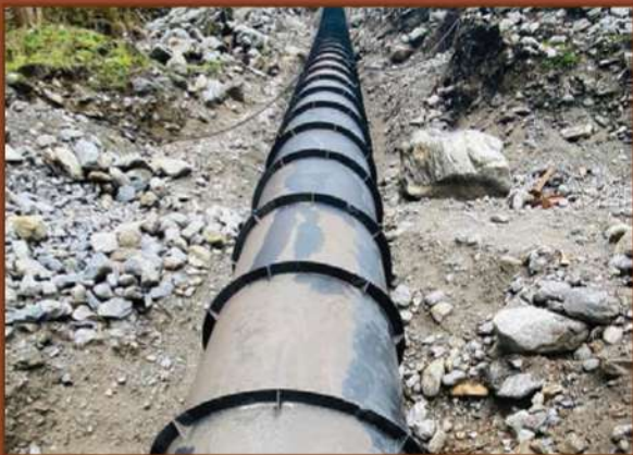
Ready to backfill
