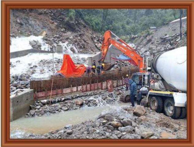
Concreting works of Flushing Canal at Nupche HWs
