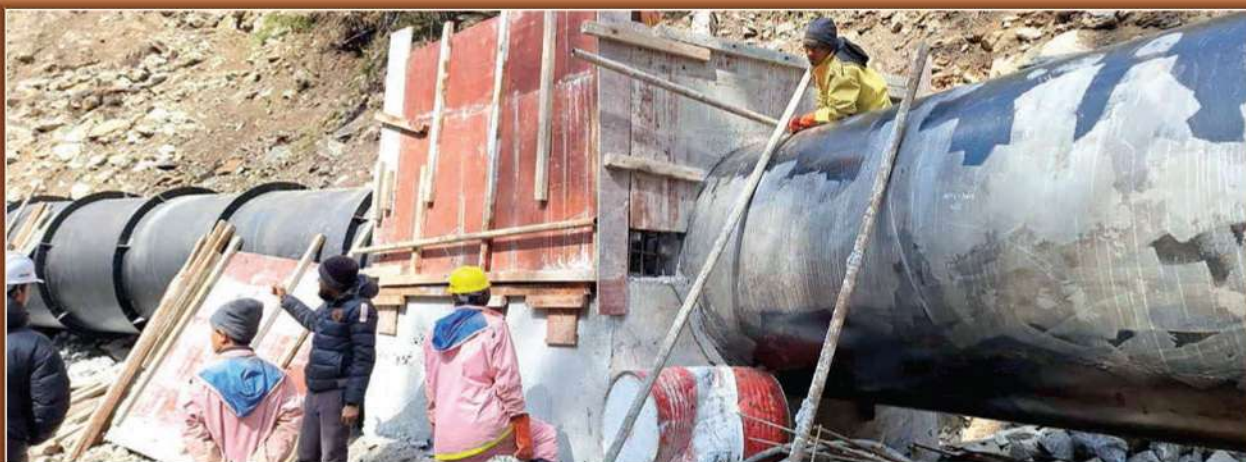
Construction of Anchor Block at Nupche HRP
