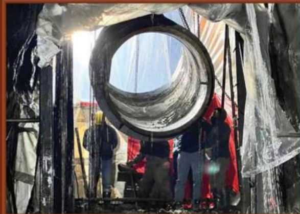
VS-2 Bend Erection works at Inclined Penstock Tunnel
