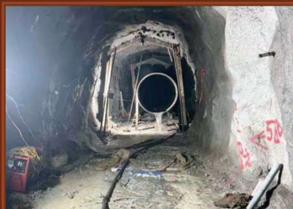
Pipe erection work in Inclined Penstock Tunnel
