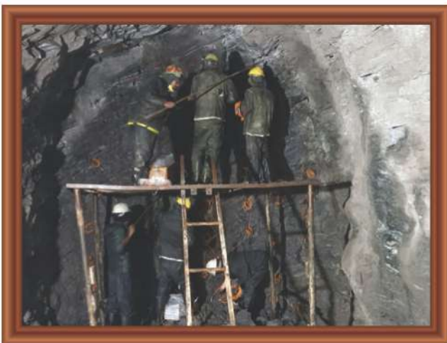
Loading explosive for blasting in tunnel
