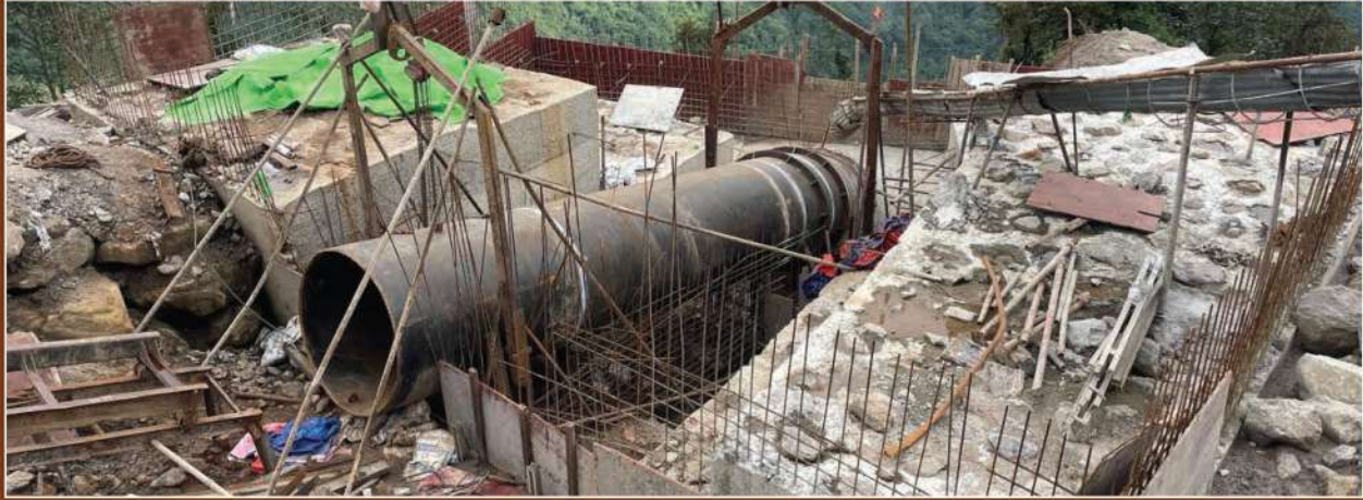
Pipe erection at Anchor Block 22
