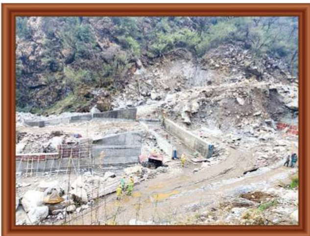
Picture showing Nupche Weir & Cut-off wall
