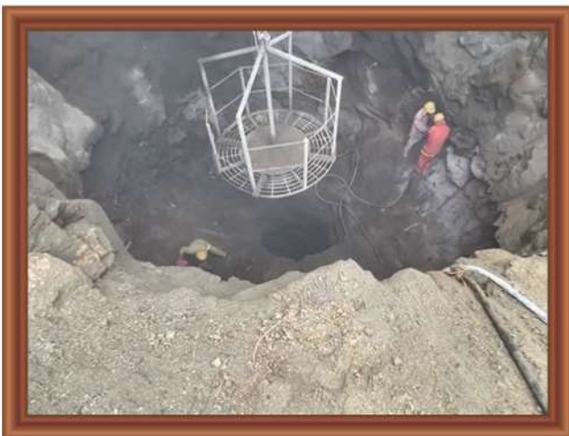
Full face excavation at Surge Shaft
