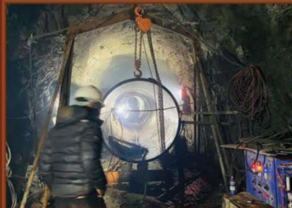
Pipe Erection works at Inclined Penstock Tunnel
