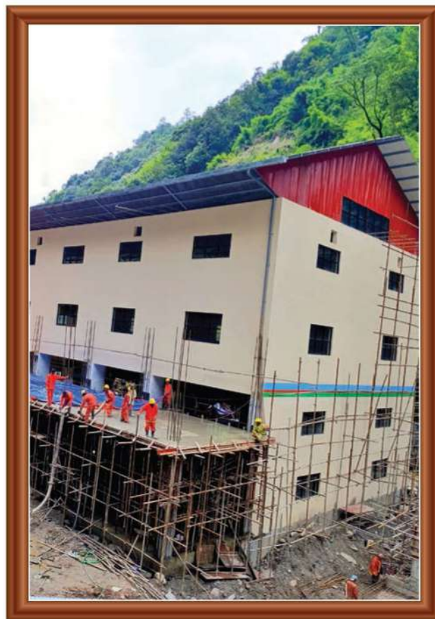
Slab casting works of control building at Powerhouse
