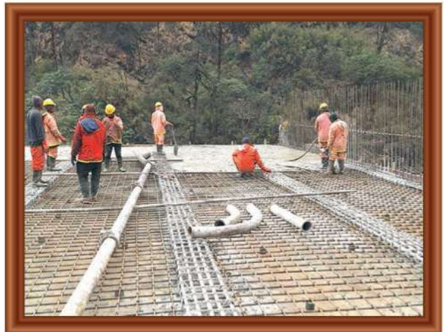
Nupche Settling Basin -Cover Slab Work
