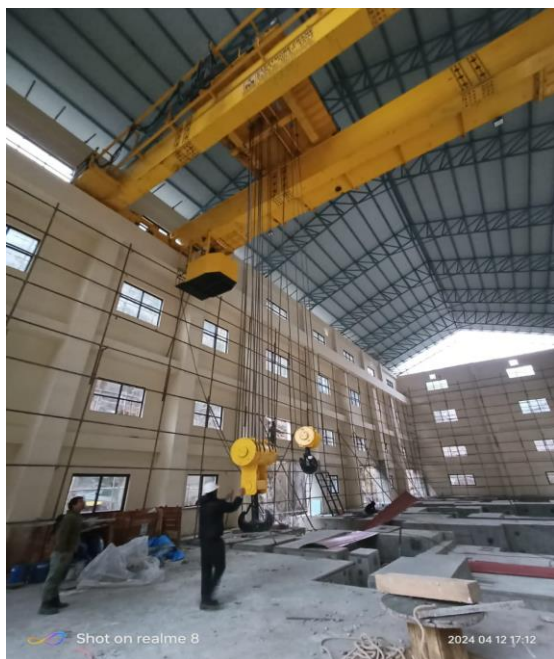
Figure showing: EOT Crane Testing and Commissioning inside Powerhouse
