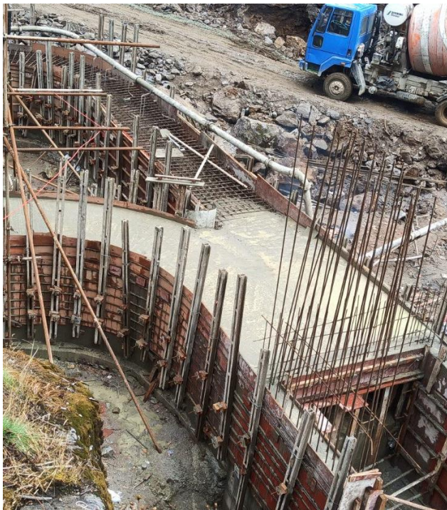
Figure: Concreting of Flushing Culvert
