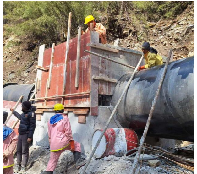
Figure: Concreting of Anchor Block along penstock pipe alignment.
