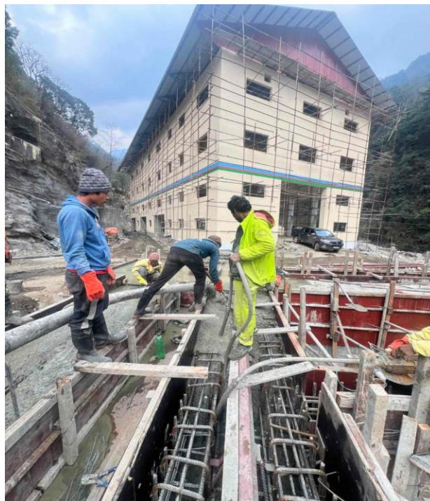
Figure:- Transformer foundation
