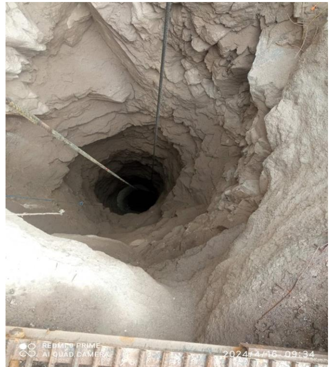
Figure: Mucking Work of Pilot Hole
