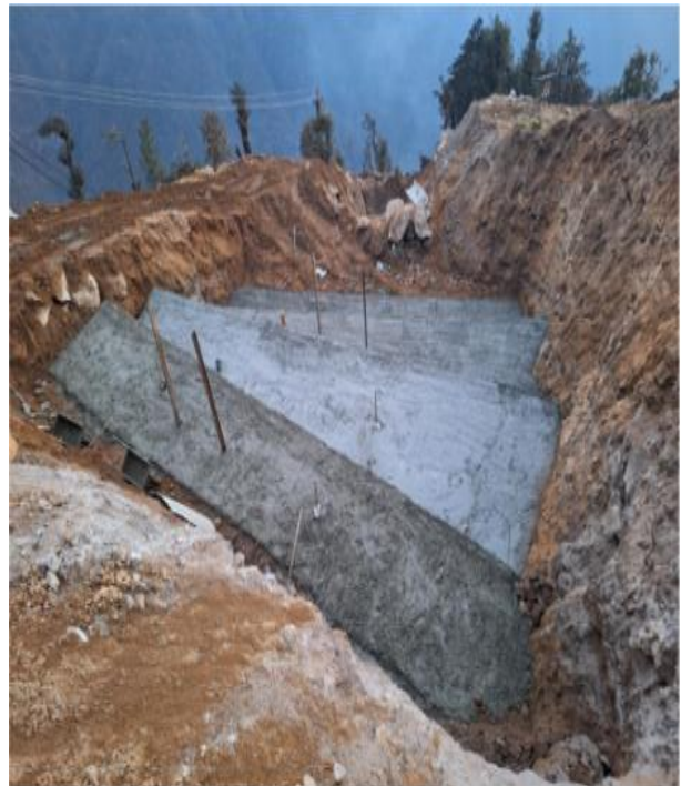
5.3: Blinding Concrete in AB-22 Penstock.
