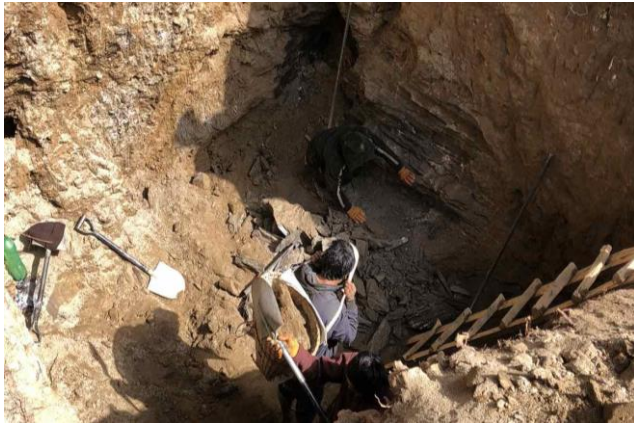
Figure: Excavation in Pit in Tower 6/2
