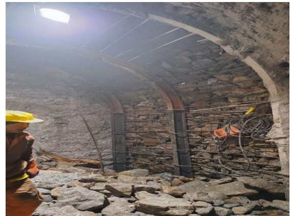
Figure: Rib Installation and stone packing at Nupche.
