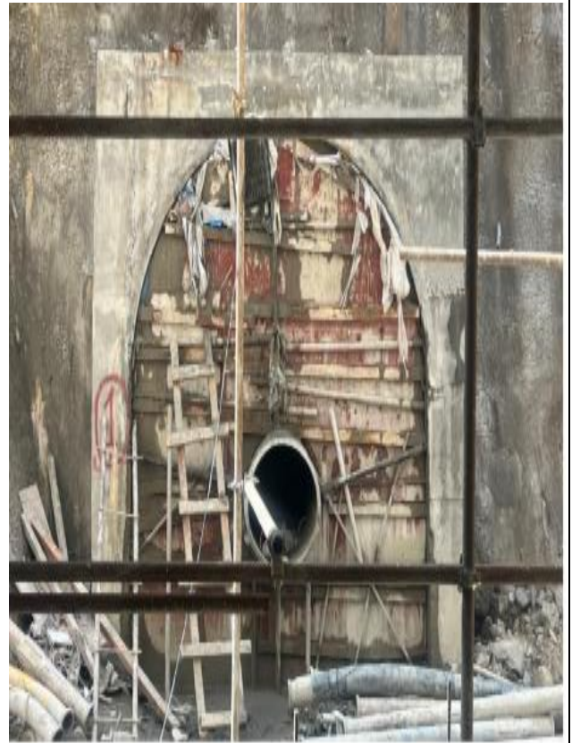
Figure: Unit 1 branch pipe concreting.
