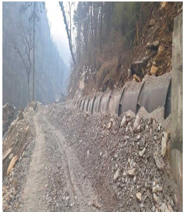
Figure: Back Filling Works
