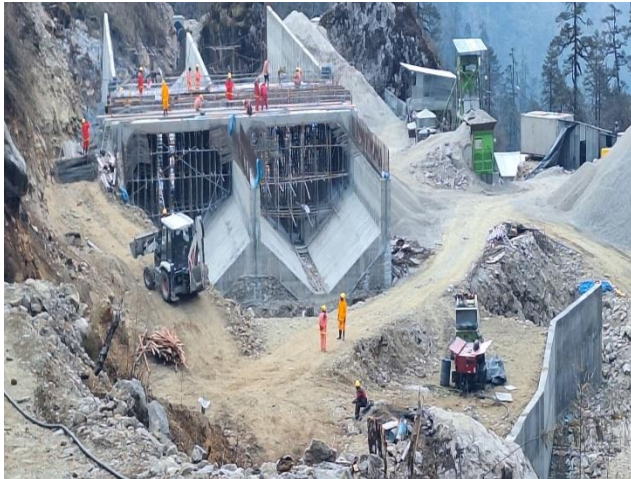
Figure: Concreting of Flushing Culvert
