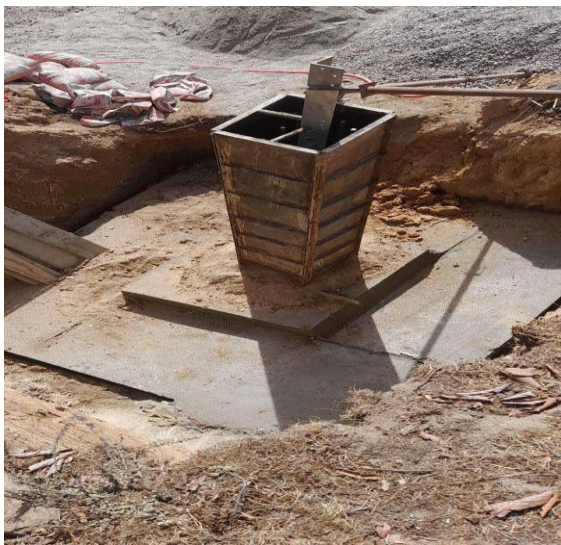
Figure: RCC in Tower Foundation with Stub
