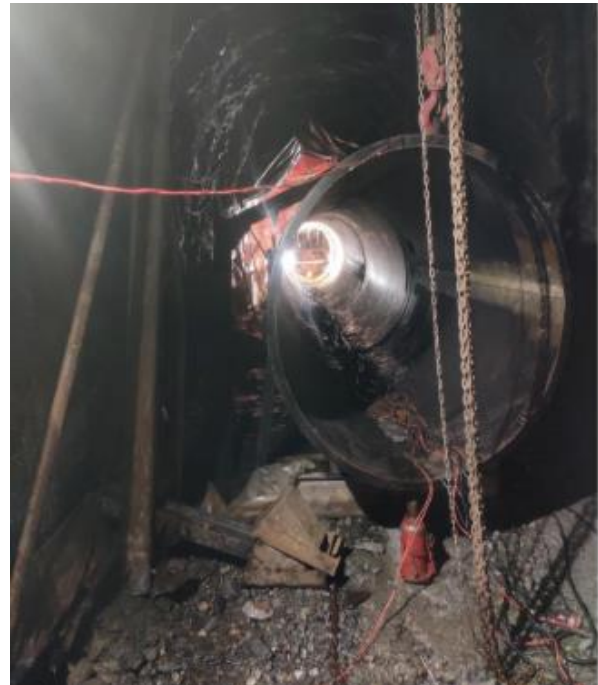
Figure: Erection of pipe at Penstock Tunnel
