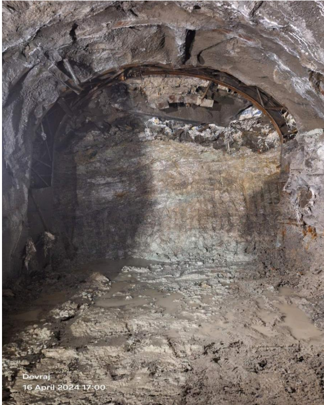
Figure: Likhu Inlet Face Stabilization
