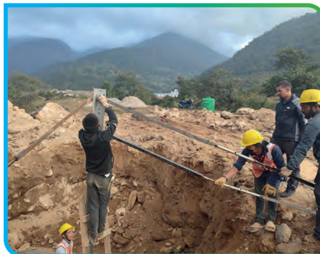
Tower Excavation works
