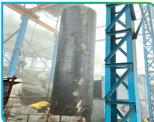
Weight Test of Penstock Pipe at Vertical Shaft
