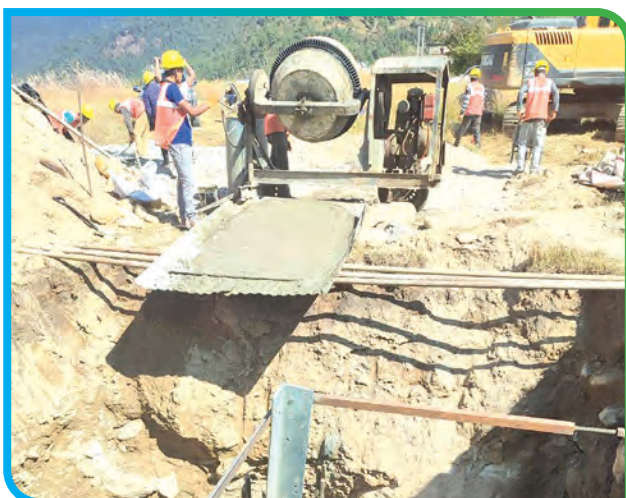
Foundation concreting works of TL Tower
