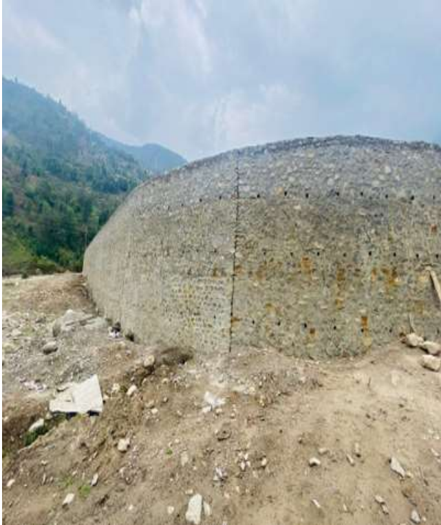
Figure: Protection structure at Garjyang Substation
