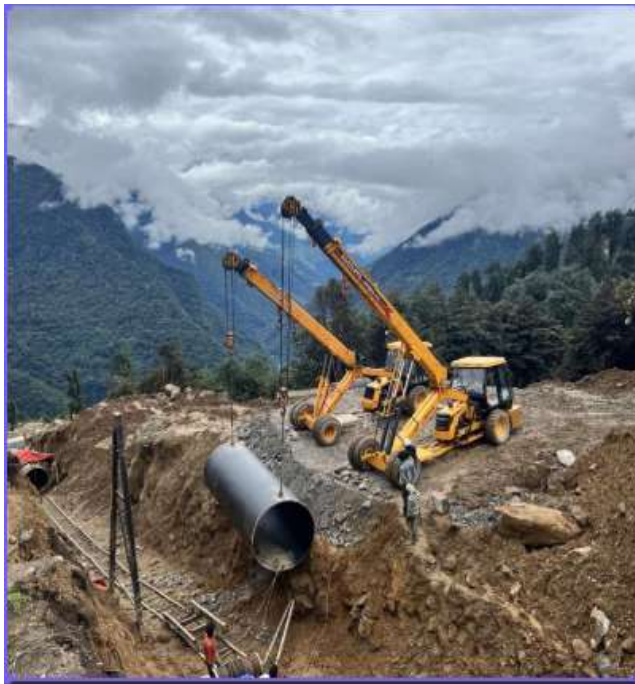
Figure: Pipe Erection Work at penstock
