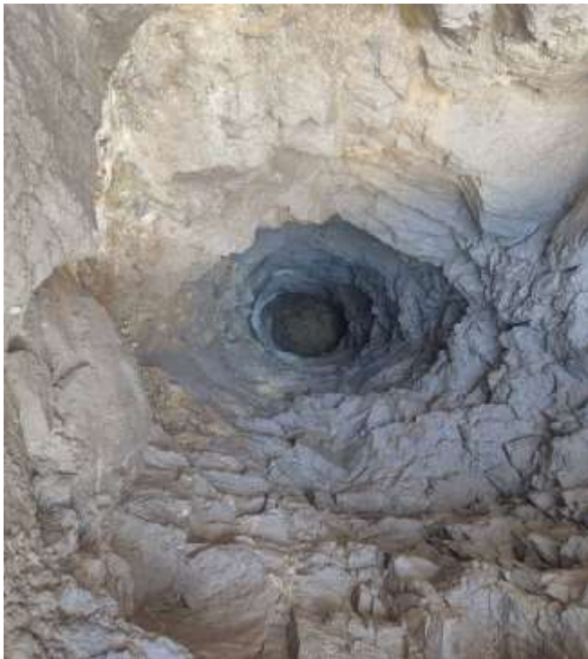
Figure: Breakthrough of Pilot Hole
