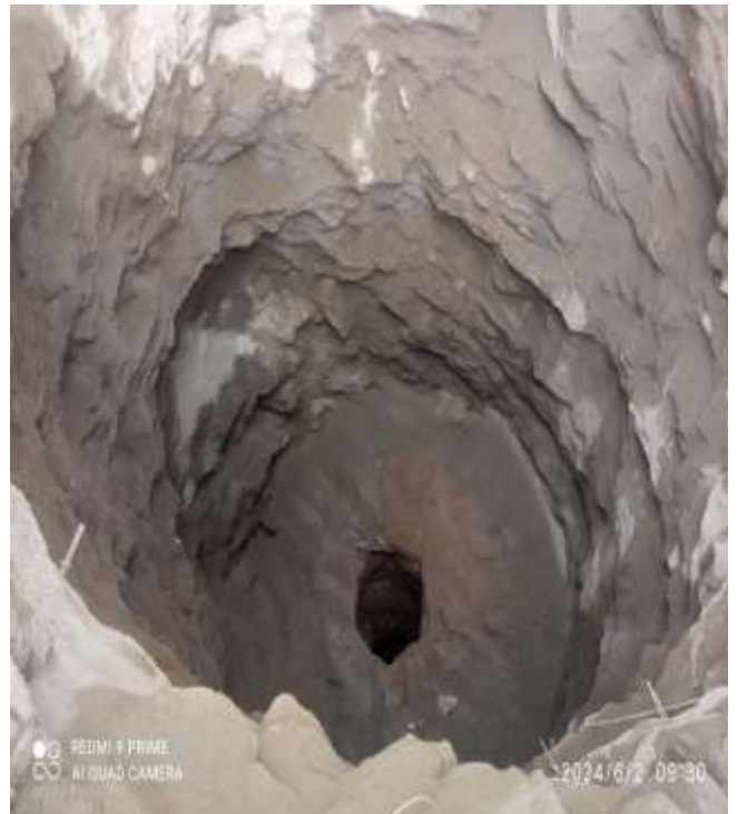
Figure: Full face Excavation work of Surge Shaft
