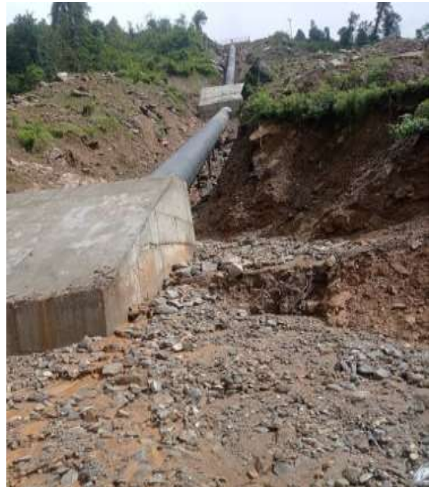
Figure: Completed section of Penstock
