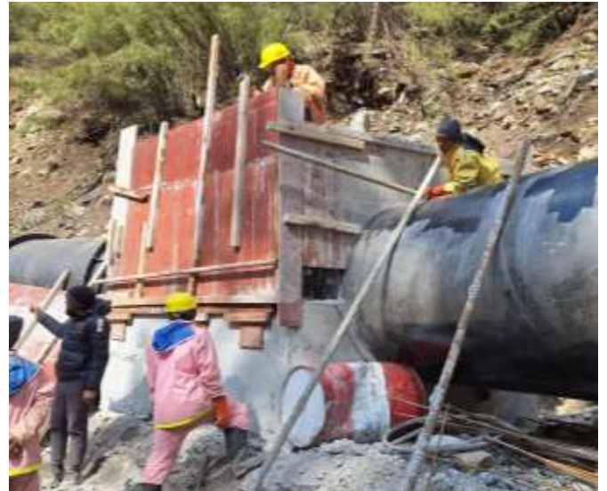
Figure: Concreting of Anchor Block along penstock pipe alignment.
