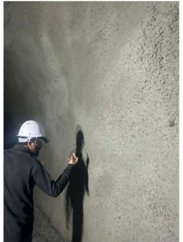
Figure: Final Shotcrete of Likhu Tunnel
