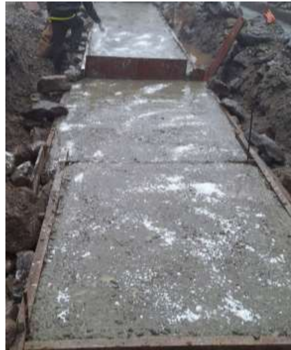
Figure:PCC at Bed Load Flushing Culvert
