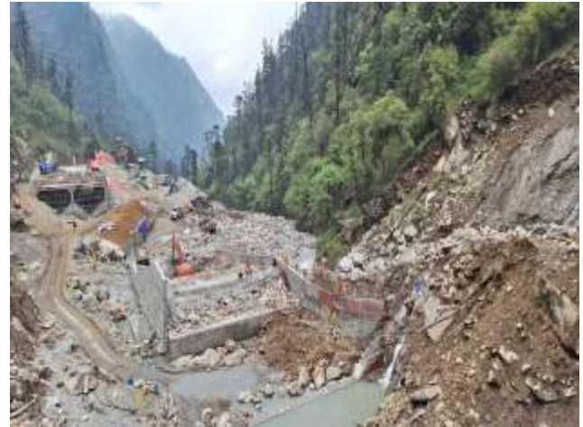
Figure:PCC at Bed Load Flushing Culvert
