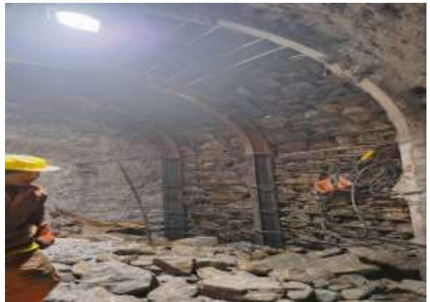
Figure: Rib Installation and stone packing at Nupche.
