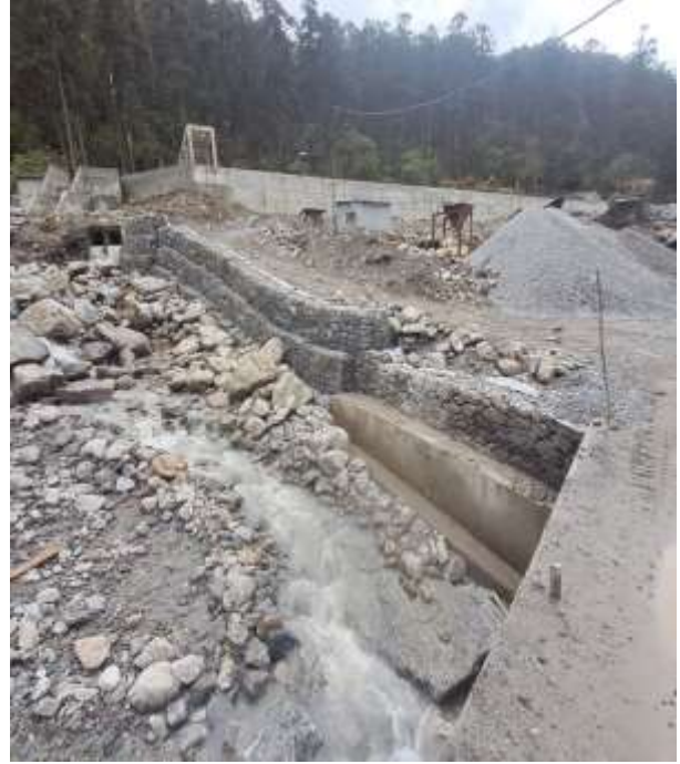
Figure Showing:- Likhu Headworks Intake Superstructure.
