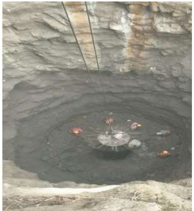
Figure: Full face Drilling and Excavation work of Surge Shaft
