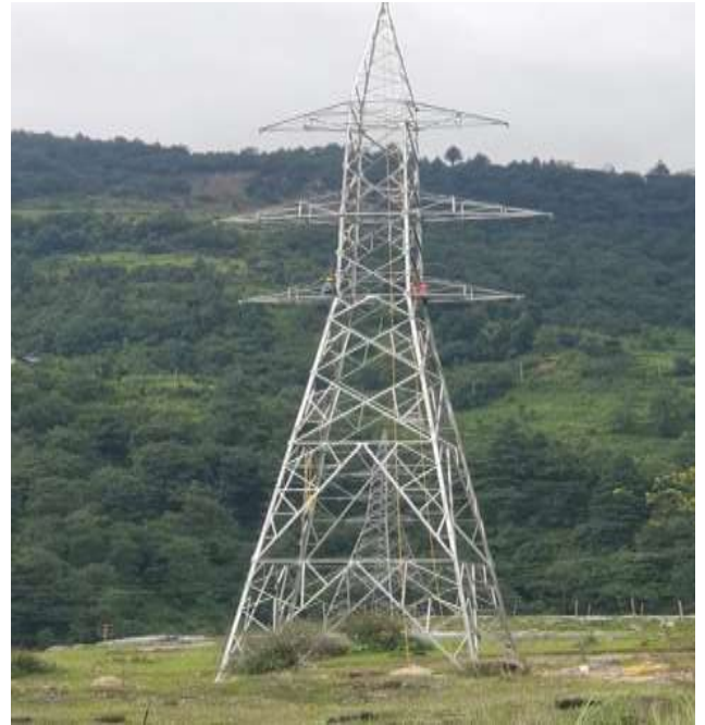
Figure: Erection of Tower AP23
