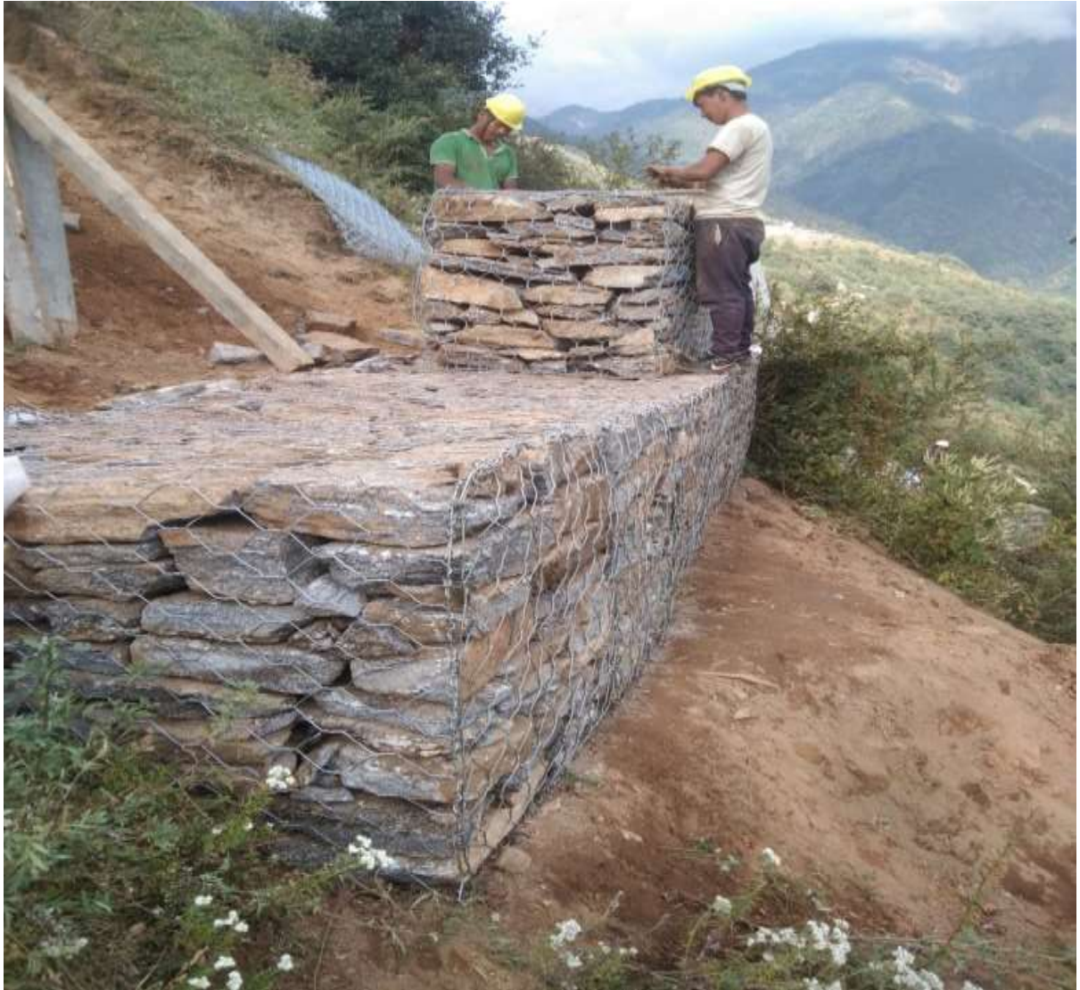
Figure: Tower Protection Works
