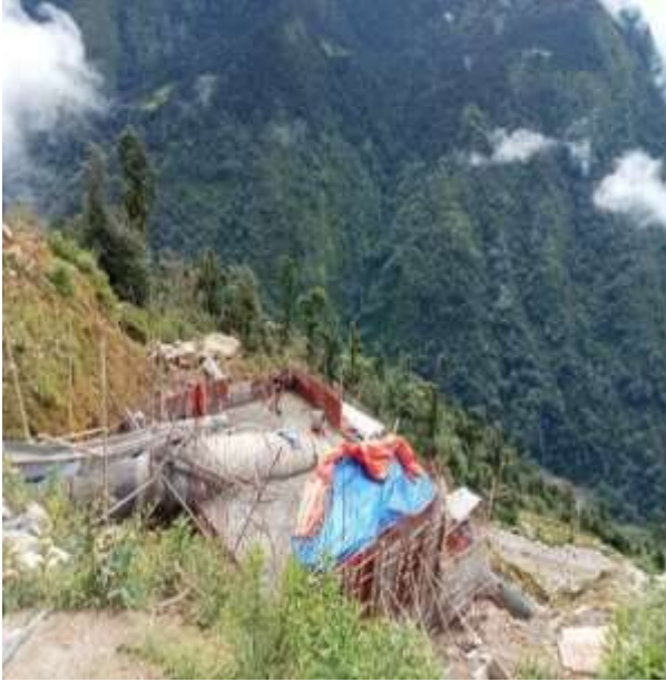
Figure: Completion of AB18 along Penstock Alignment.
