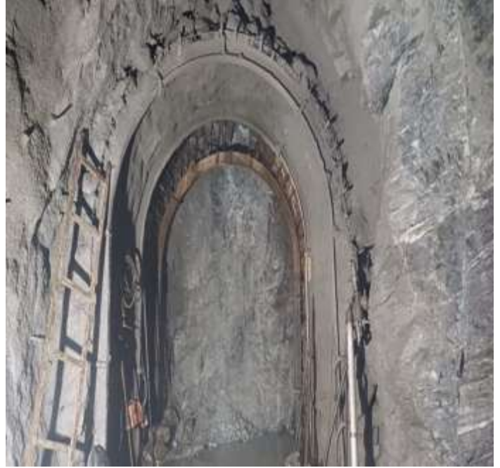
Figure: Rib Installation at Nupche Inlet at 0+814m
