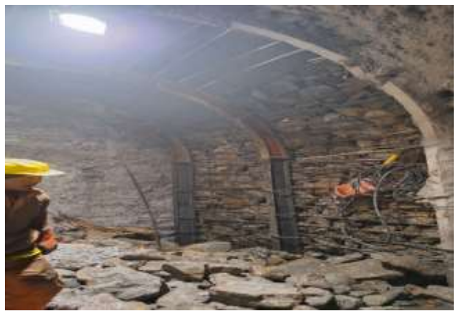
Figure: Rib Installation and stone packing at Nupche HRT.
