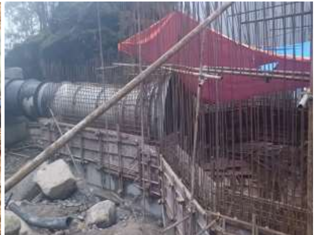
Figure: Nupche Headworks installation of Bellmouth and Concrete works.
