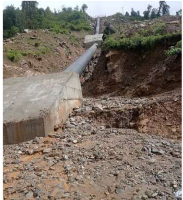
Figure: Completed section of Penstock
