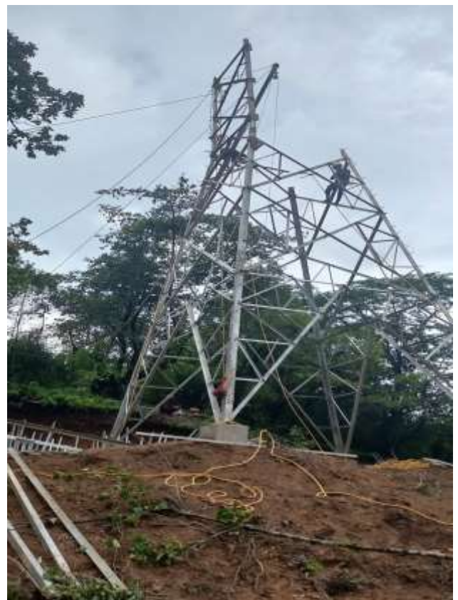
Figure: Erection of Tower AP23
