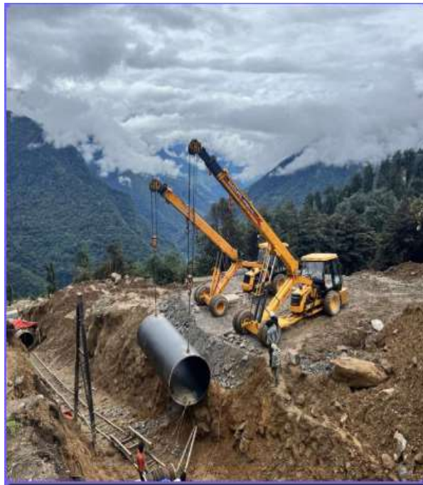
Figure: Pipe Erection Work at penstock.
