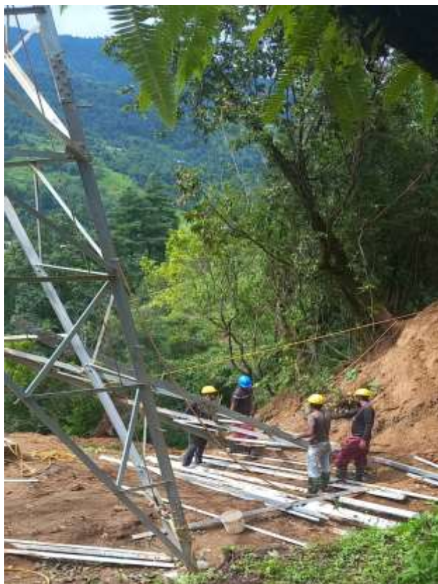
Figure: Erection of Tower AP23
