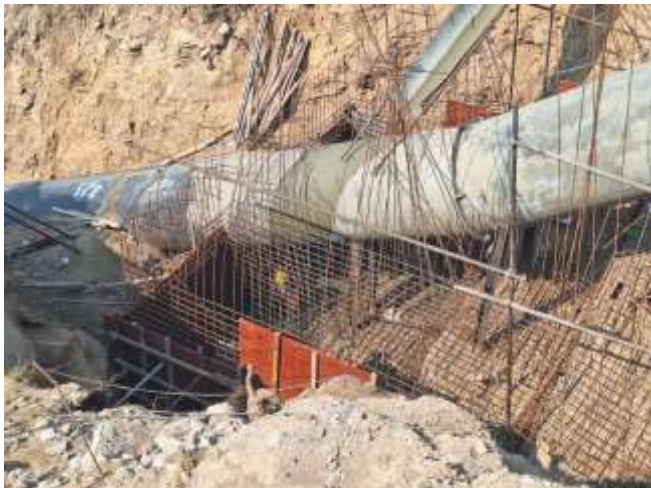
Figure:-Concreting of Anchor Block along penstock alignment.
