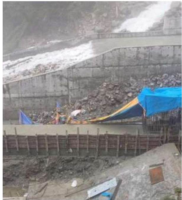
Figure: Water flowing through main weir and Concreting of Gravel Flushing at Nupche HWs.
