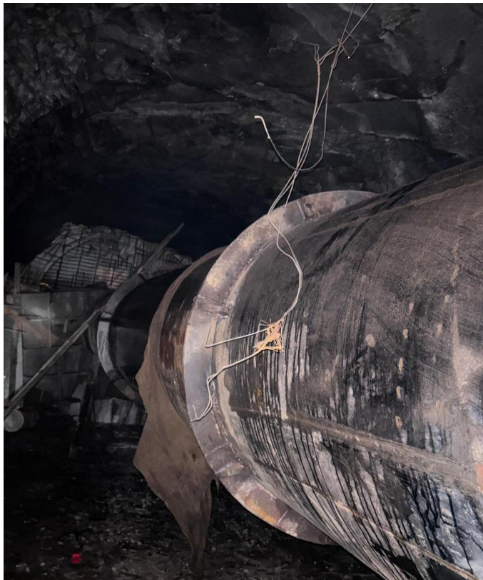
Stiffener welding at PT
