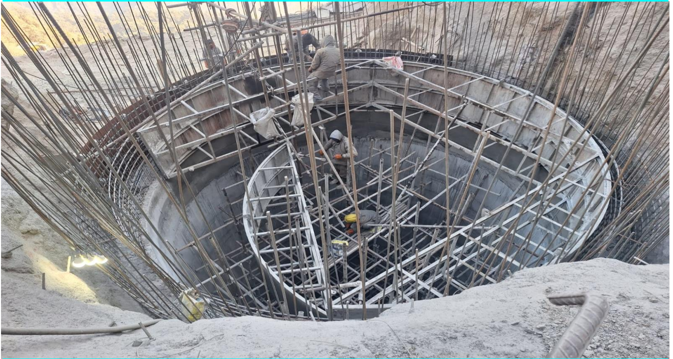
Formwork at Surge shaft
