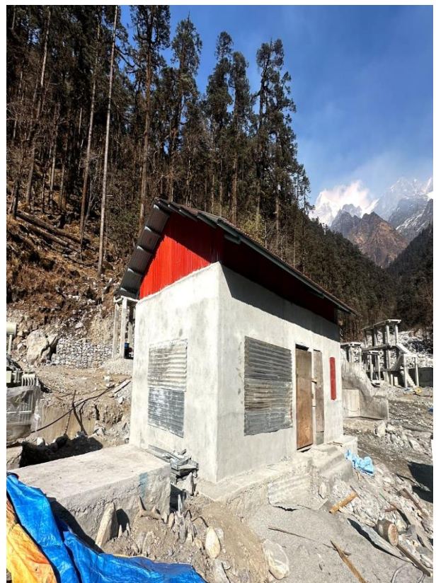
Likhu Headwork Control Building
