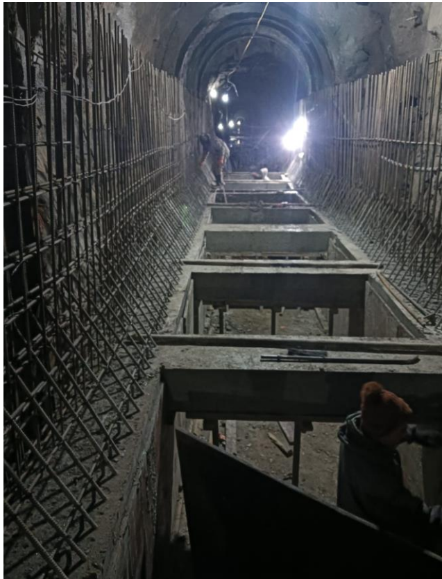
Concreting at Rock Trap
