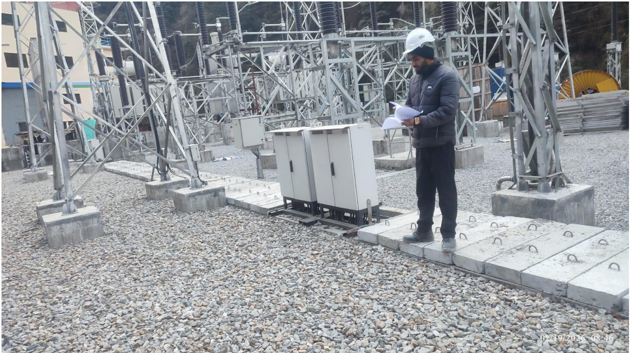
Ongoing Inspection Work
