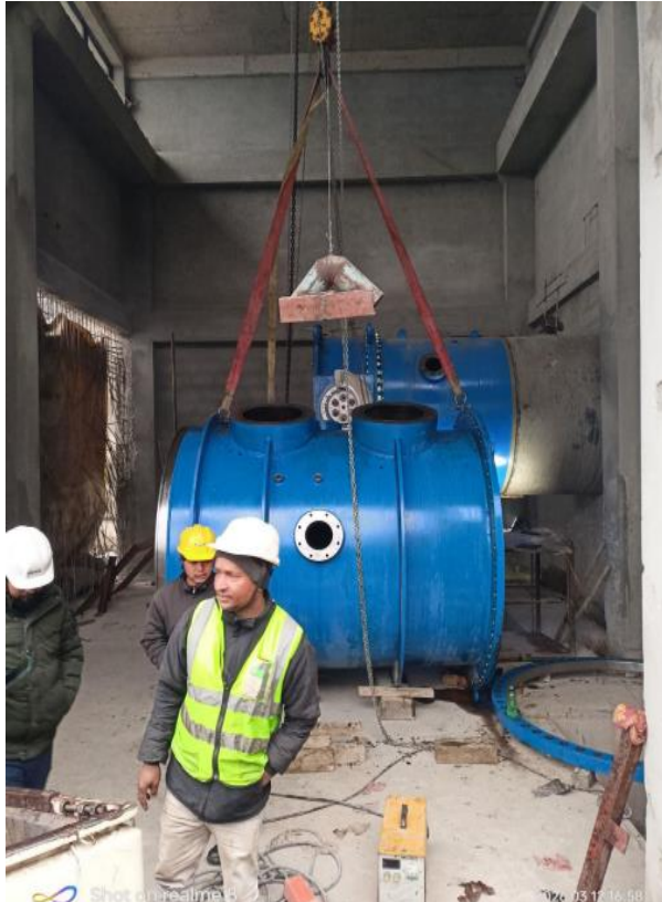
PPV installation Ongoing
