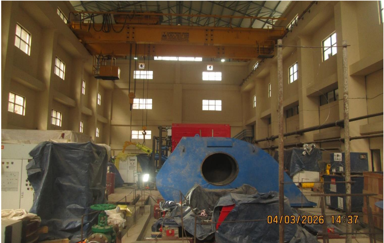
Installation of 3 rd Turbine Housing
