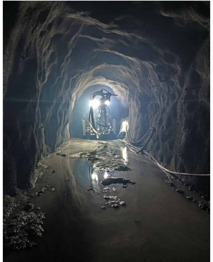
Shotcrete works currently in progress
