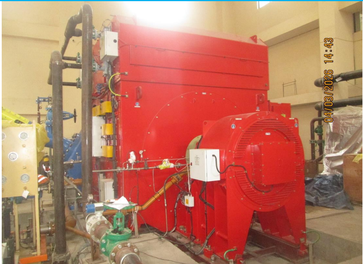
Complete Installation of 2 nd Generator
