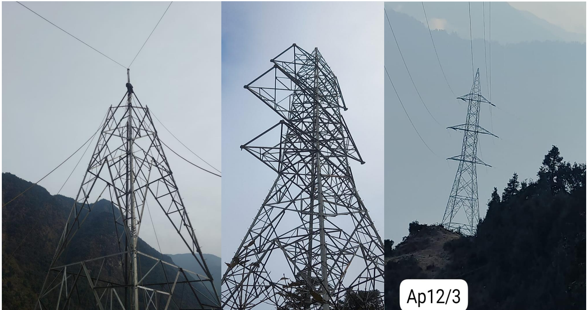
Ongoing works of Transmission Line.
