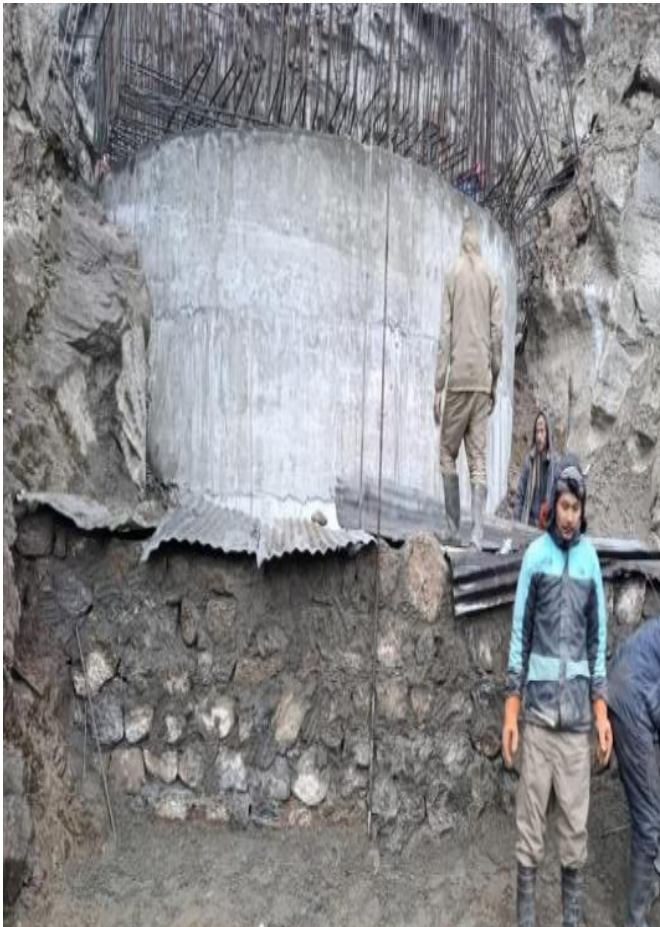
Stone masonry at the Surge shaft at Ground level
