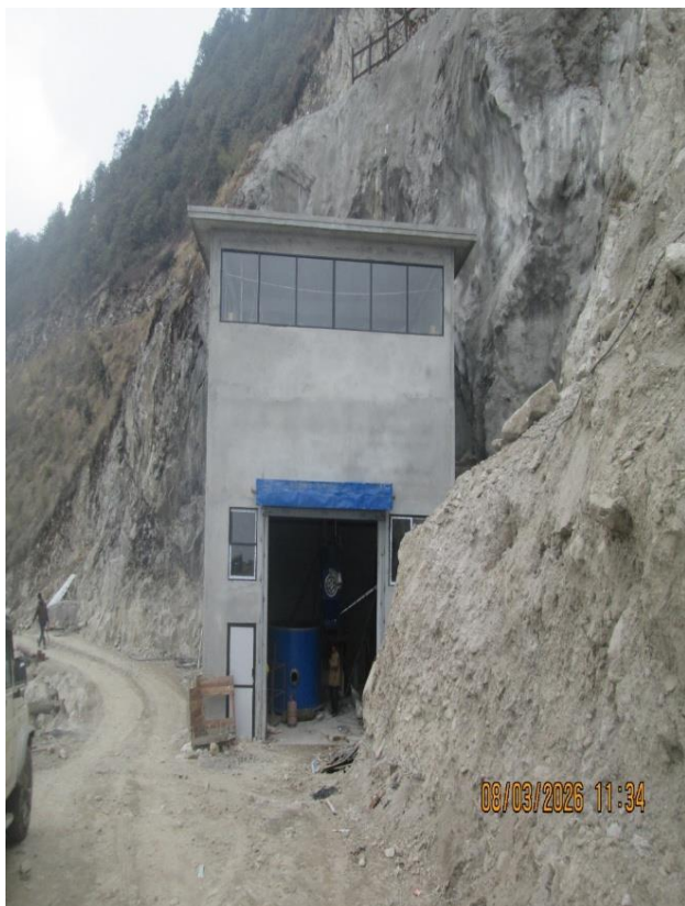
PPV House after Completion
