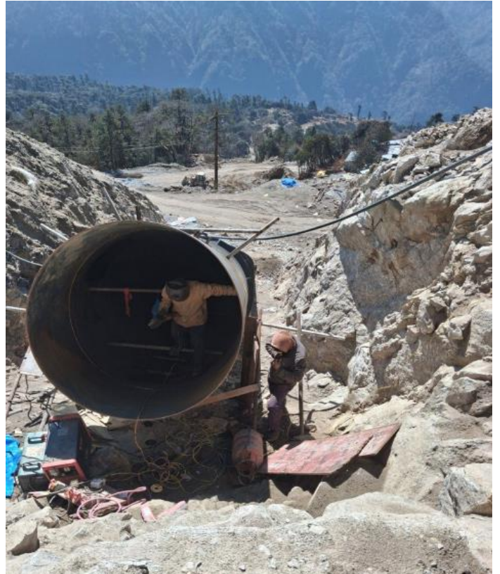
Welding works at Penstock Pipe
