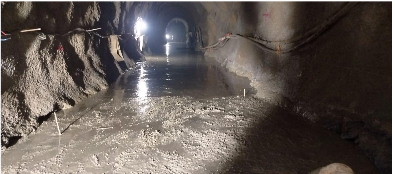
Ongoing Invert Lining Concreting
