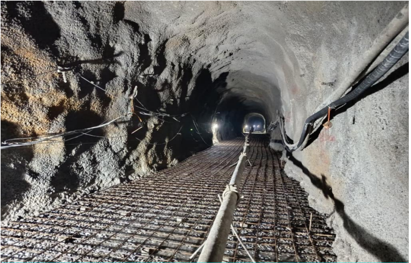
Rebar work for Invert Lining
