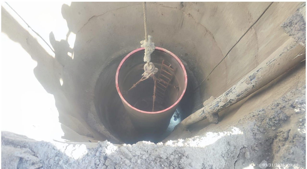
Concreting at VT
