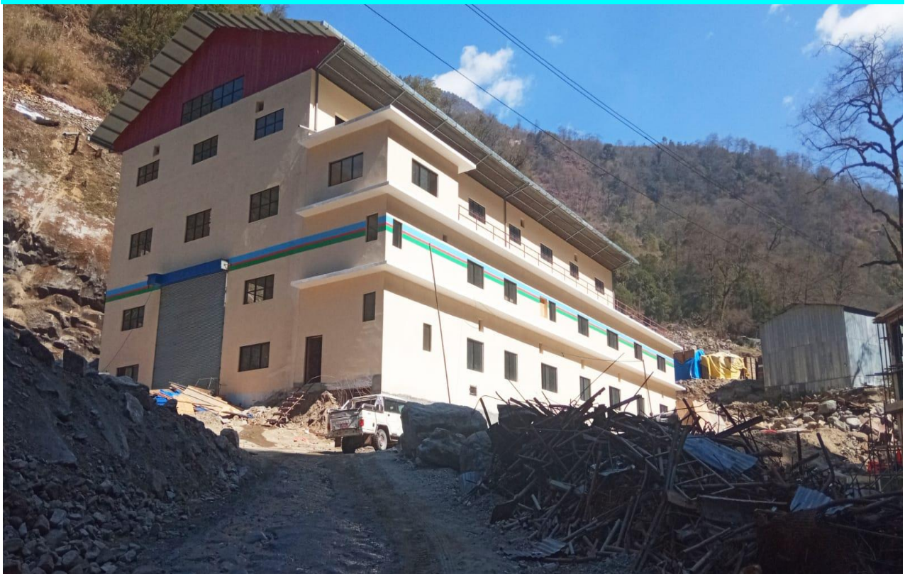
Work Progress in Powerhouse
