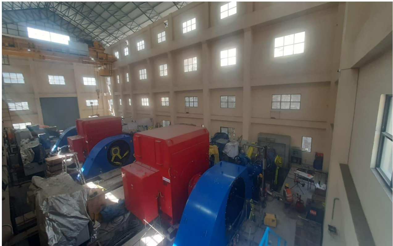
Overview of Completed Unit 1 and Unit 2
