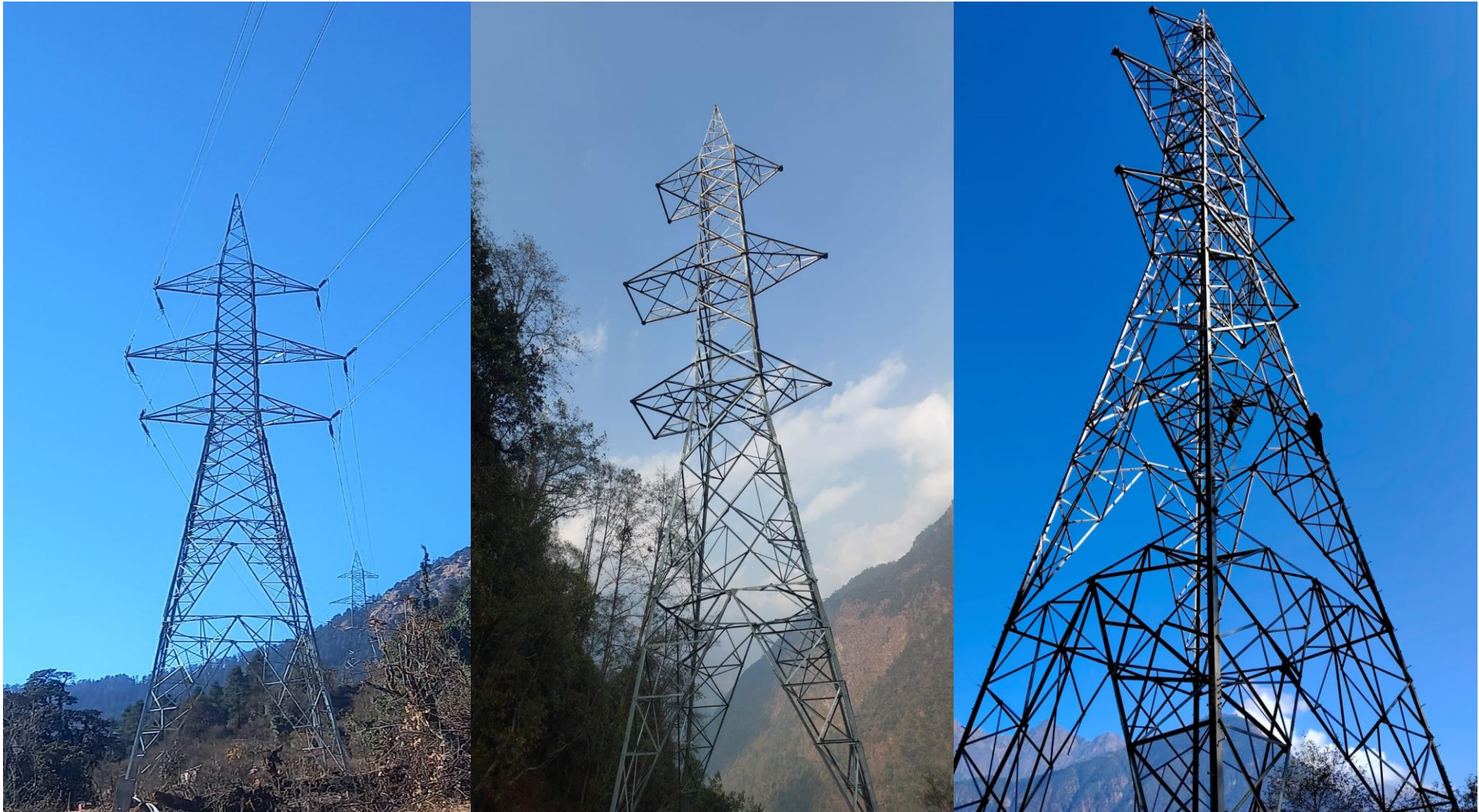
Ongoing works of Transmission Line.
