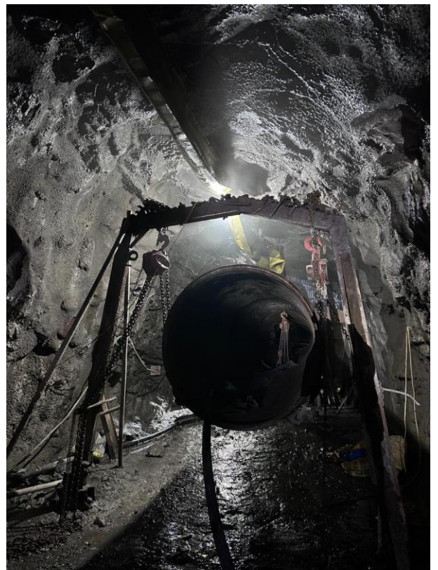
Pipe erection at PT
