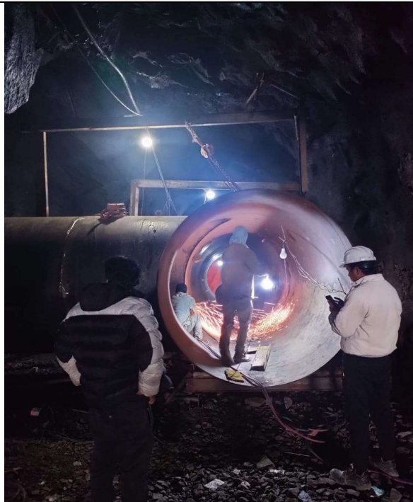
Fig-12: Pipe Erection work at Outlet Tunnel (T-junction to connecting tunnel)
