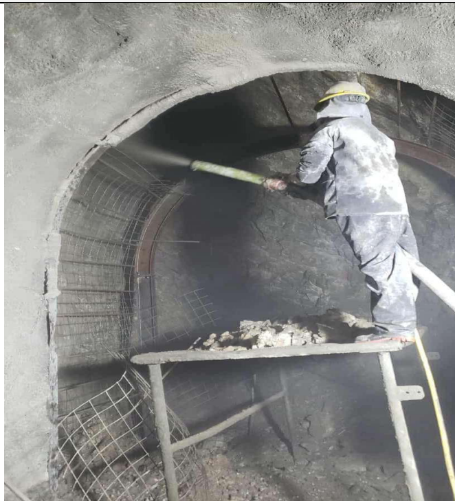
Fig-16: Support works(shotcrete) at Rib section in tunnel
