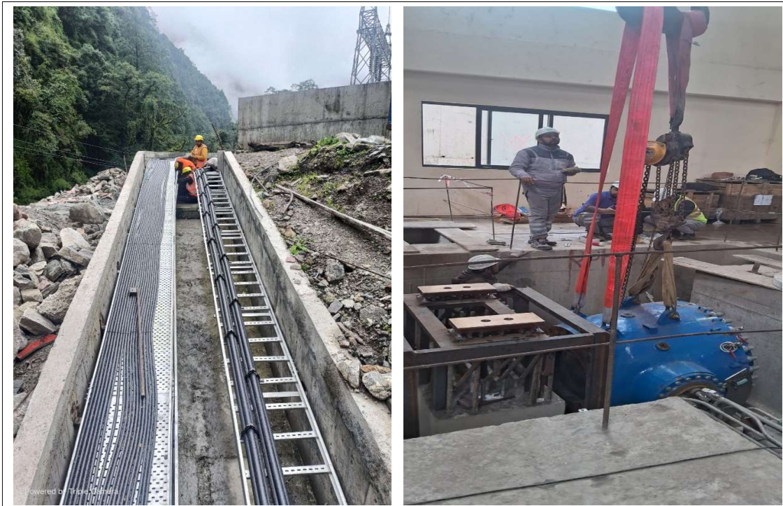
Fig-5 Power cable Dressing at Switchyard (Electromechanical Works)
