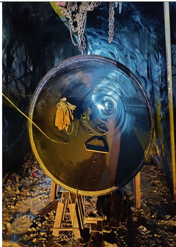
Fig-9: Pipe Erection work at Inclined Penstock Tunnel
