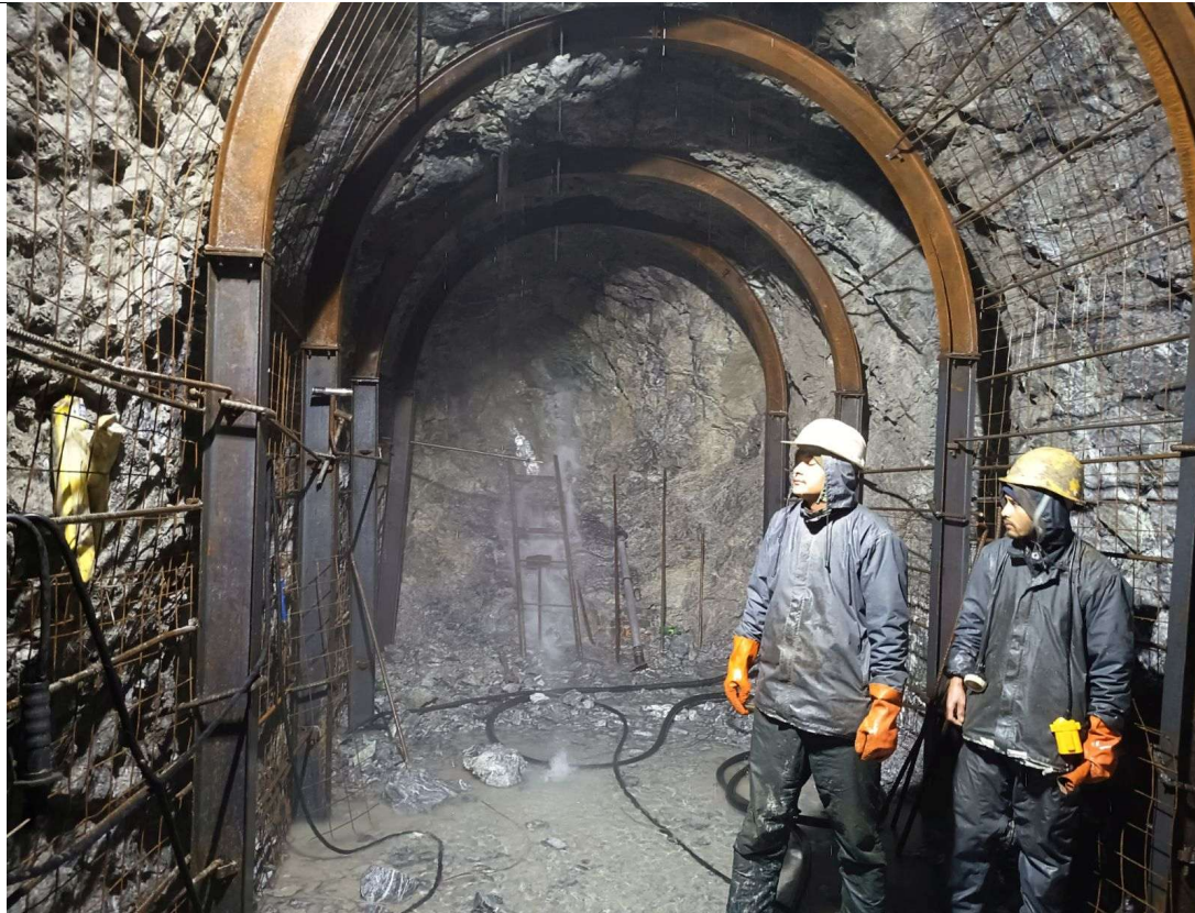
Fig-13: Installation of Rib support at Adit (F7) D/S tunnel face
