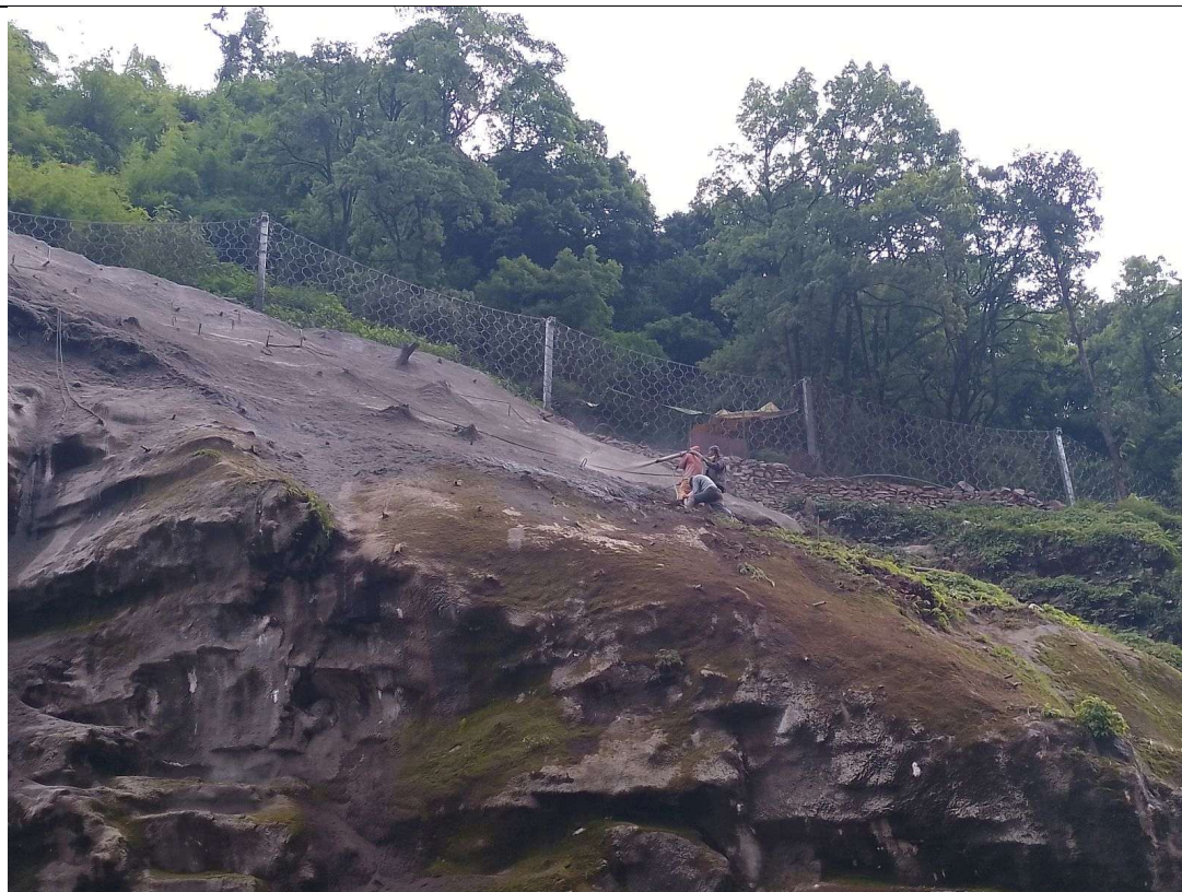
Fig-7: Installation of Rock fall Net for powerhouse Protection
