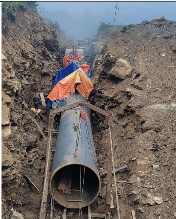
Fig-10: Penstock Pipe Erection Work from AB26 D/S)
