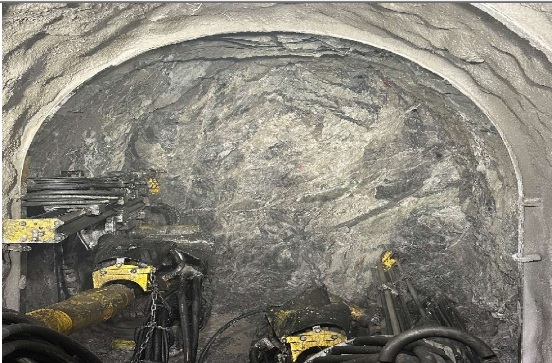
Fig-14: Face Drilling by Boomer at Outlet (F8) HRT
