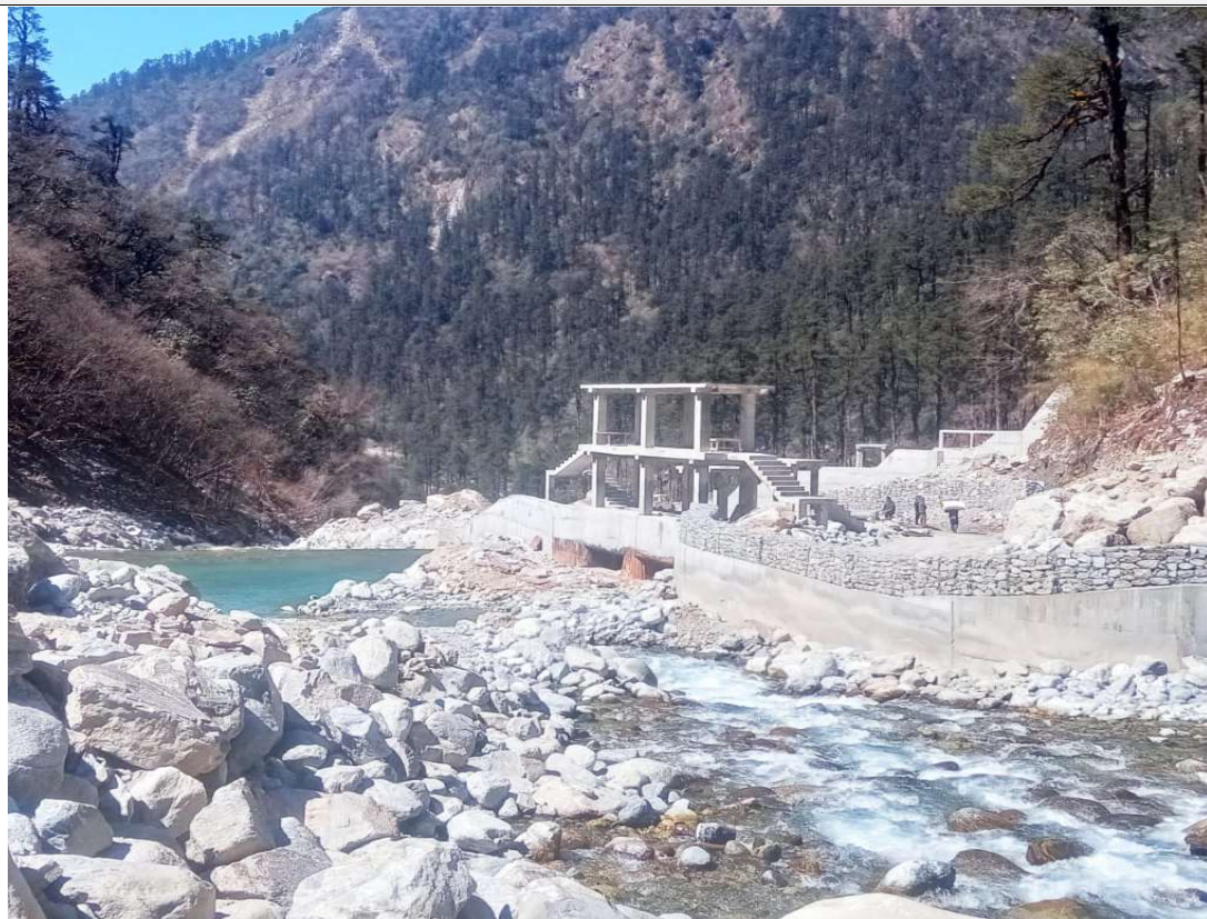
Fig-20: Overview of Completed Weir/Intake of Likhu Headworks
