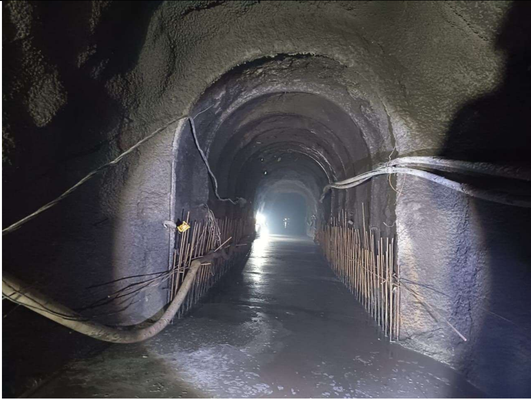
Fig-15: Invert Lining at Invert of Likhu(face-4) Tunnel
