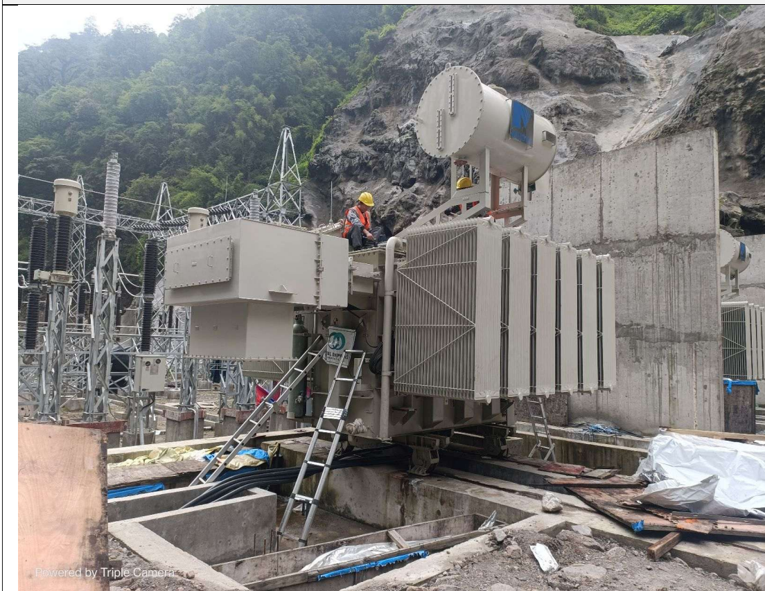
Fig-6: Transformer Accessories Erection at Powerhouse (Electromechanical Works)
