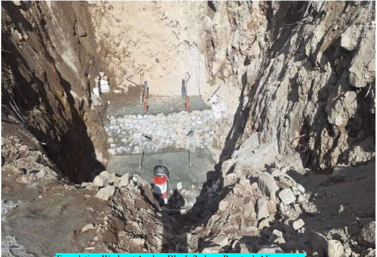
Foundation Works at Anchor Block-2 along Penstock Alignment.
