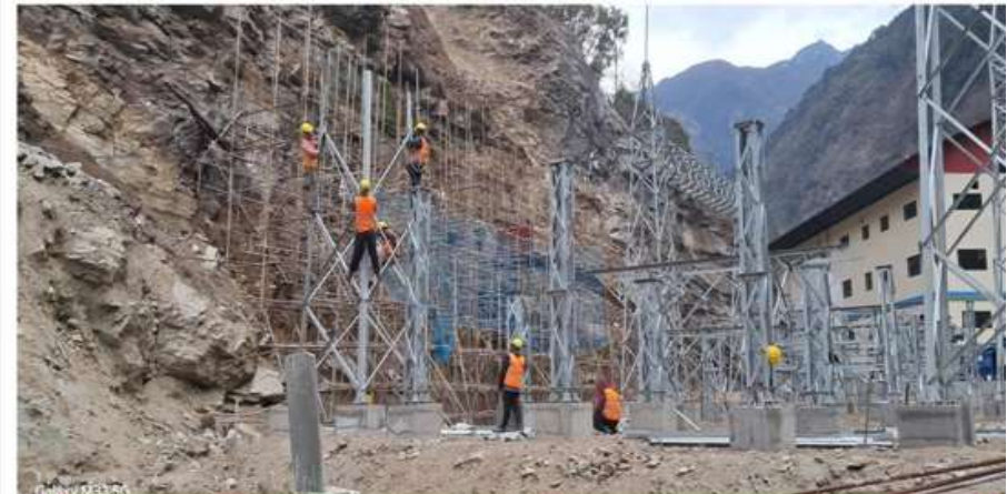
Switchyard Gantry Erection Works.
