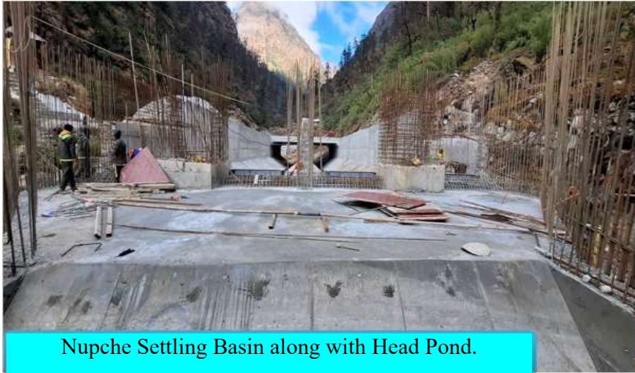
Concreting at Forebay Head Pond top column at Nupche Headworks
