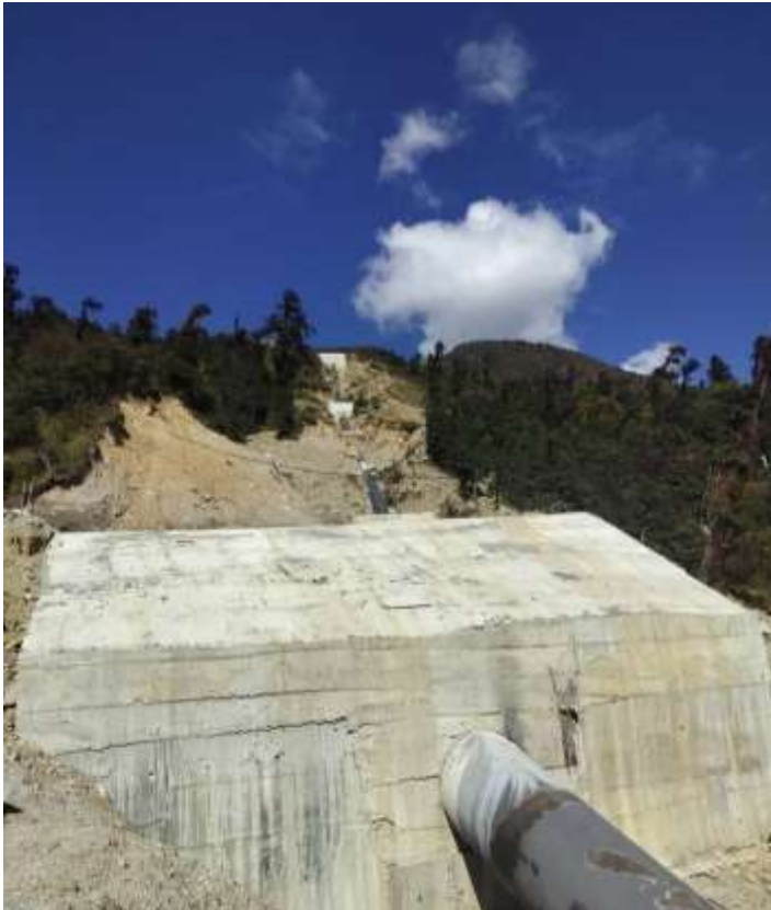
Completed Anchor Blocks along Penstock Alignment
