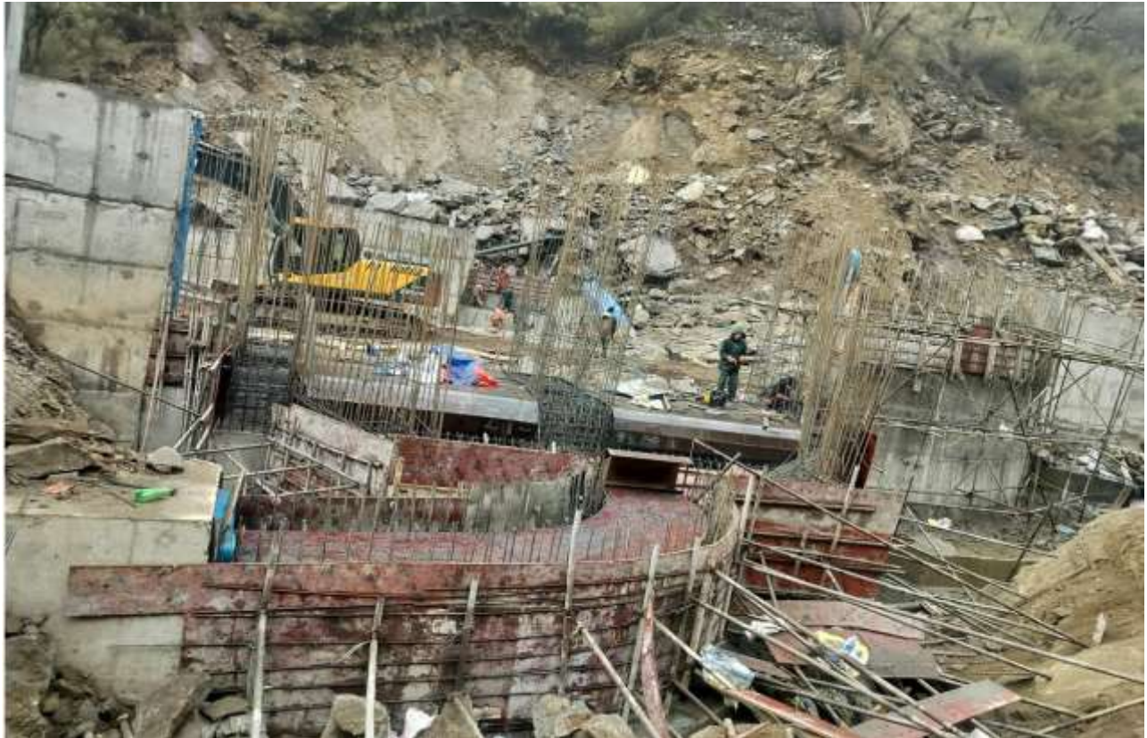
Rebar Works at Gravel Flushing and Intake.
