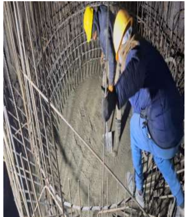
Concreting Works at Surge Shaft
