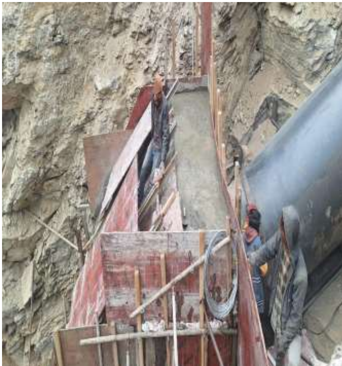
Concreting Works at AB-26 at Penstock Alignment.
