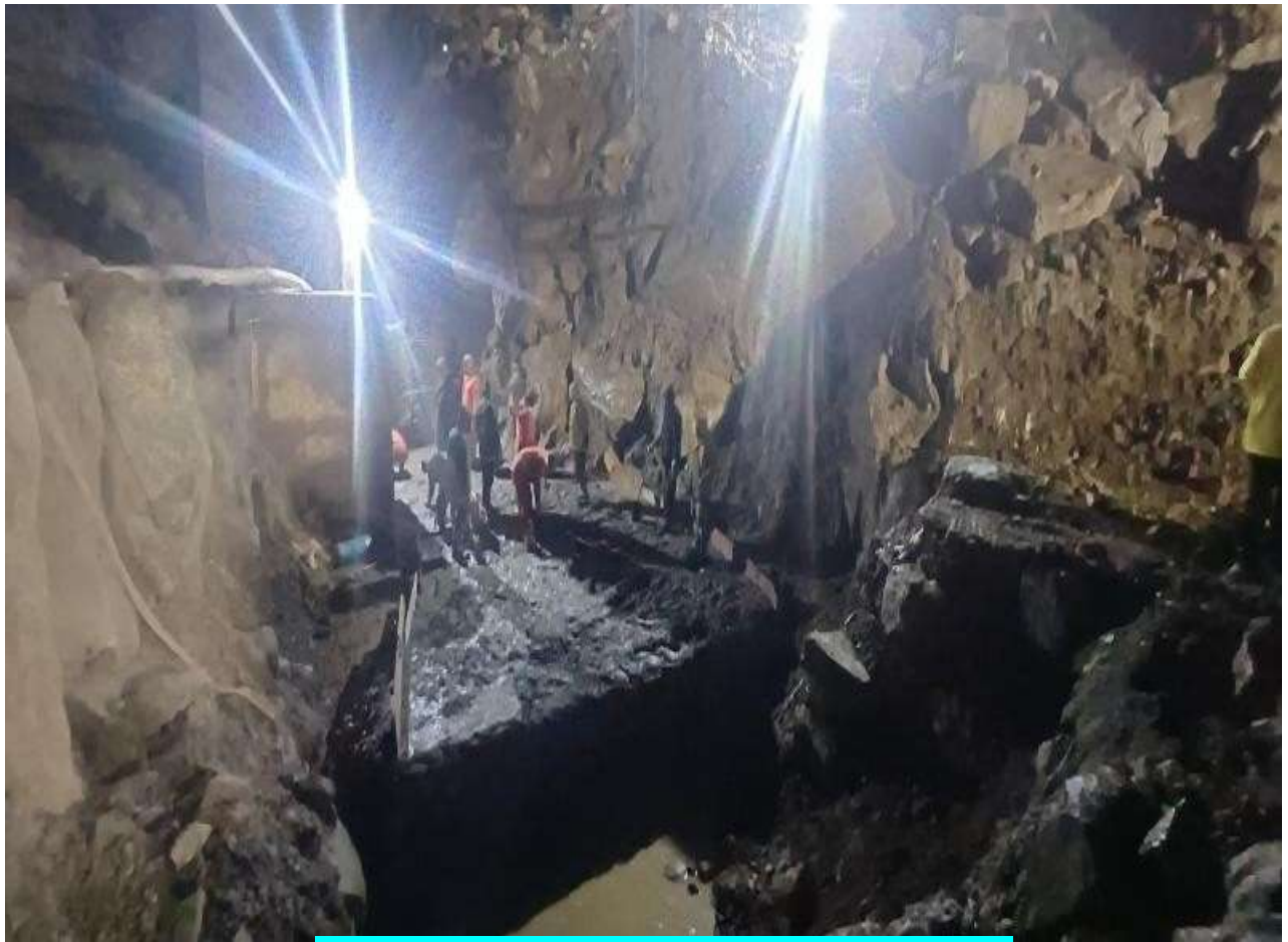
Concreting Works at Powerhouse Tailrace Area
