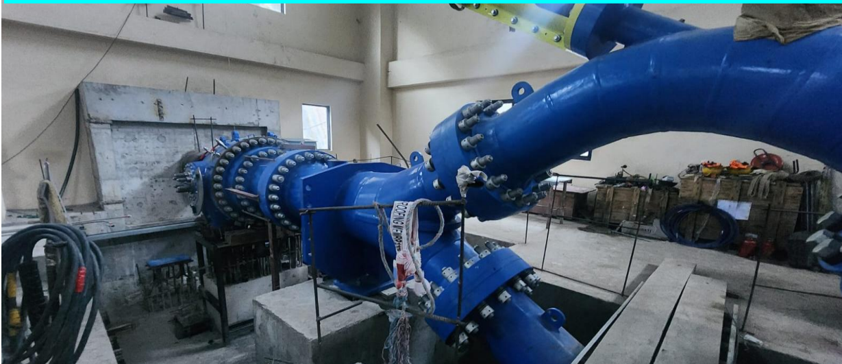
MIV alignment with Turbine Bifurcation
