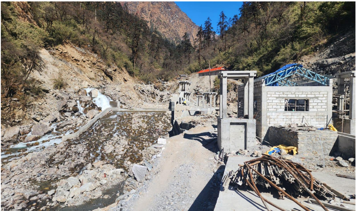
Weir at Nupche Headworks
