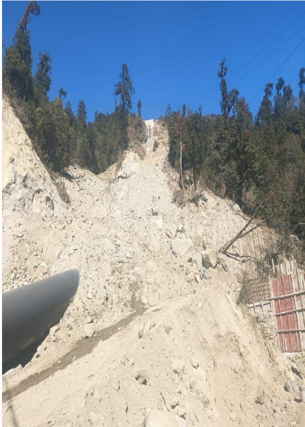
Excavation at Kholsi in P/s Alignment
