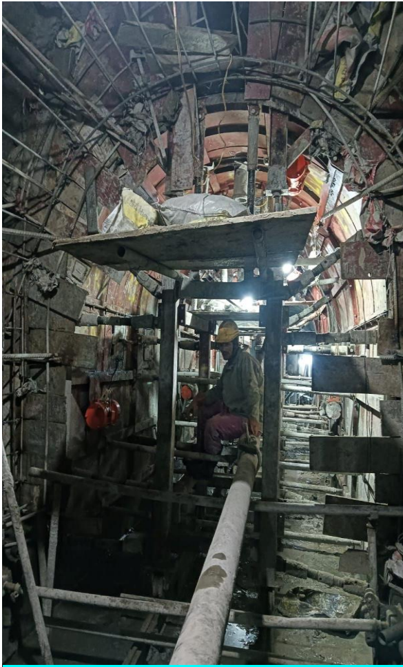
Concreting work at outlet
