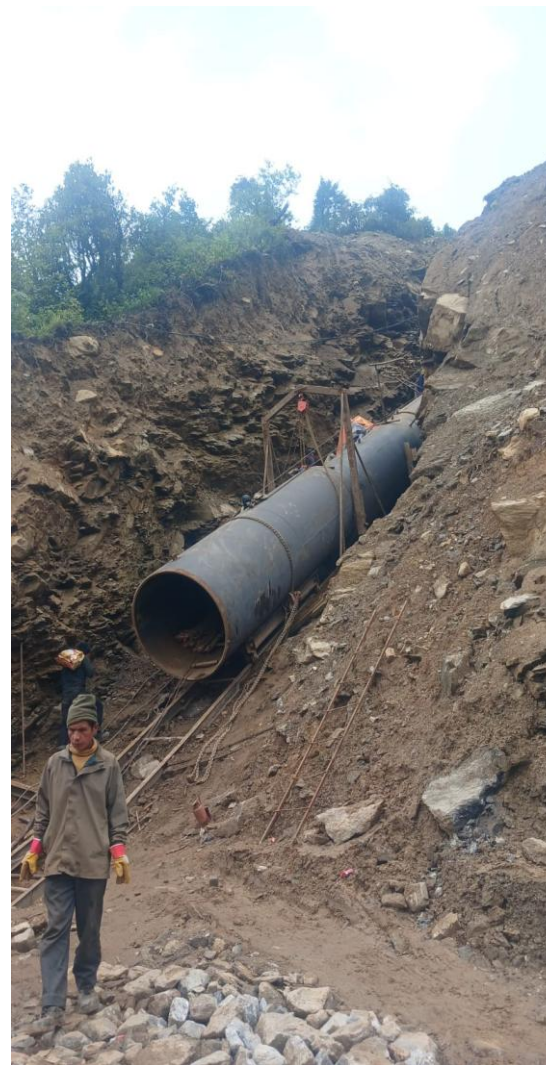
Installation of Pipe at AB26-AB27
