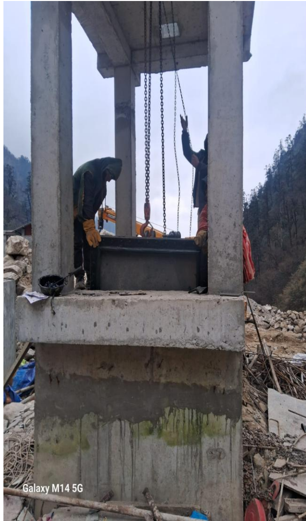
Gate Lowering at Nupche Gravel Flushing
