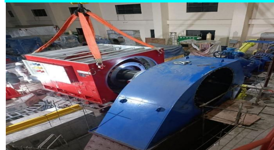
Erection of Generator
