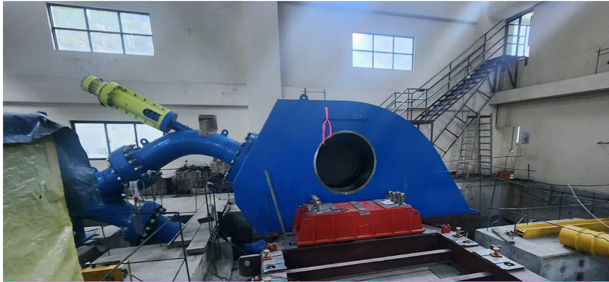
Installation of Turbine Housing
