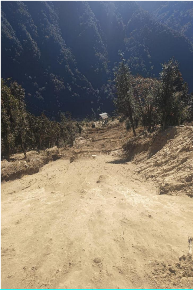
Backfilling Work along Penstock alignment
