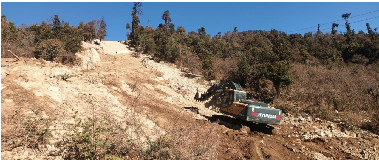
Backfilling work at Penstock alignment
