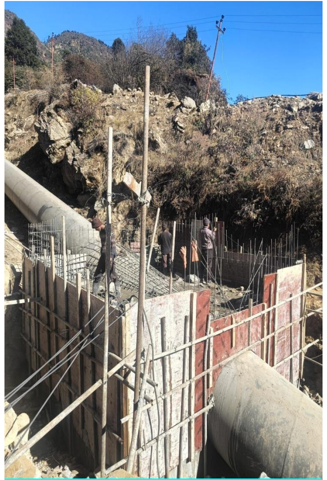
Anchor Block Concreting
