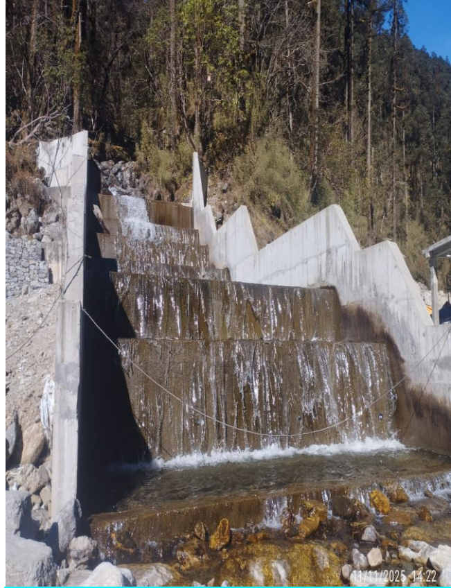
Kholsi at Likhu Headworks
