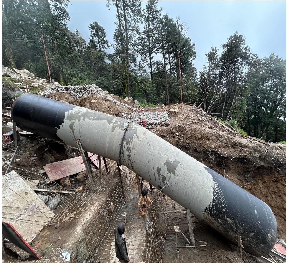
Application of Cement Latex before Concreting.
