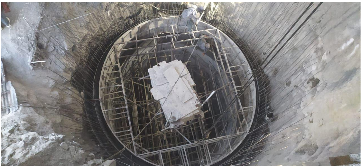
Rebarwork at Surge shaft
