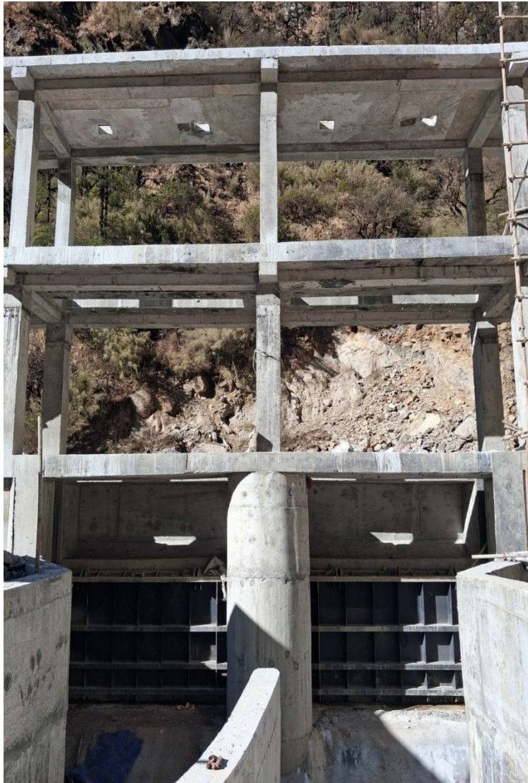
Gate Works at Likhu Intake
