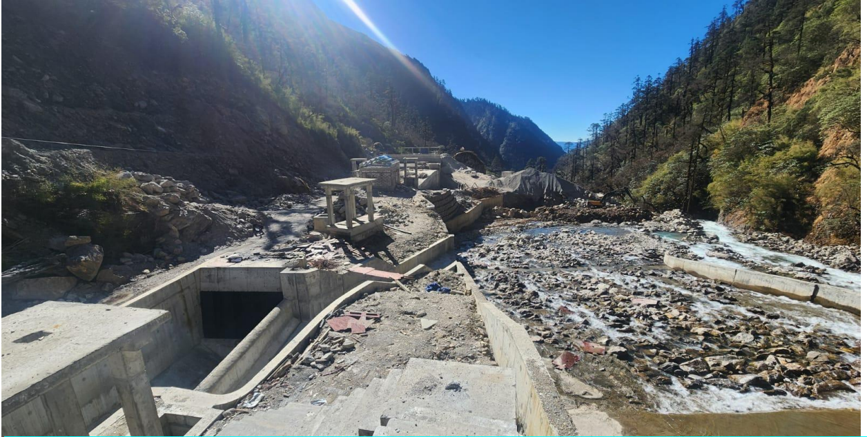
Overview of Nupche Headworks area.
