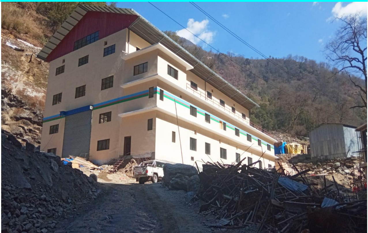
Work Progress in Powerhouse
