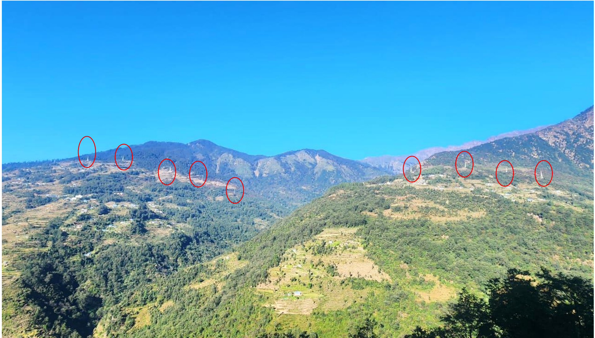
NLHP Transmission Line Towers at Kyama and Gumdel Village.
