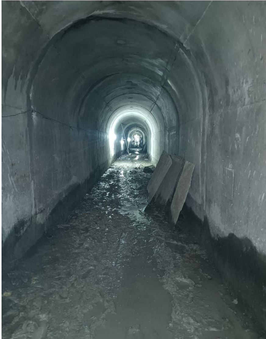
Full Lining at Headrace Tunnel (Outlet)
